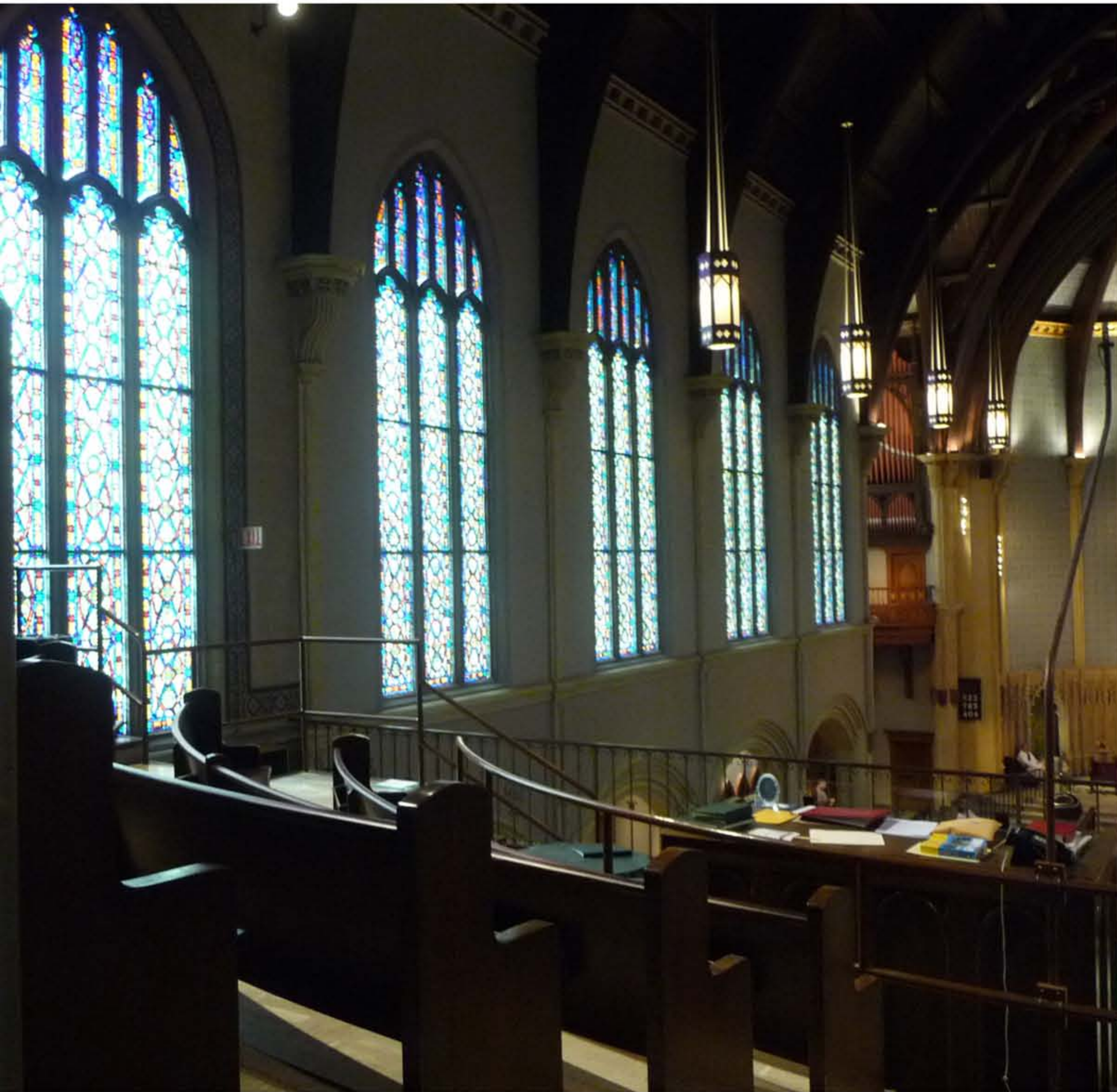
Direct Sunlight on East Sanctuary Windows-8:30am
