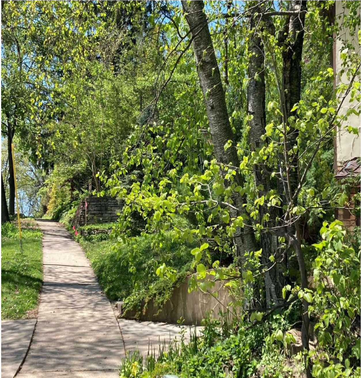
Figure 29 View from in front of 1806 Summit Ave, up the hill toward Ely Pl. You can see the survey flags marking the Applicant's narrow strip of property, but the stone retaining wall behind the flags belongs to the Morehouse House.
