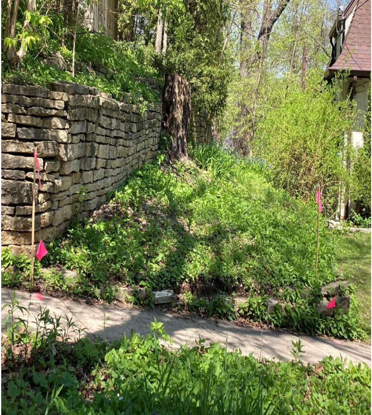
Figure 30 View from Summit Ave, looking toward N Prospect Ave. The pink survey flags on left and right mark the 10-foot-wide strip of proposed Lot 2 that extends for 55 feet to Summit Ave. The stone retaining wall to the left is not part of the Applicant's property; it is part of the landmark Morehouse House. You can also see that the lot line on the right adjacent to 1806 Summit Ave almost abuts the house. Any route of vehicular travel on this strip would endanger the house and excavation would compromise the historic stone wall of the Morehouse House. Note the mature walnut tree in the background.
