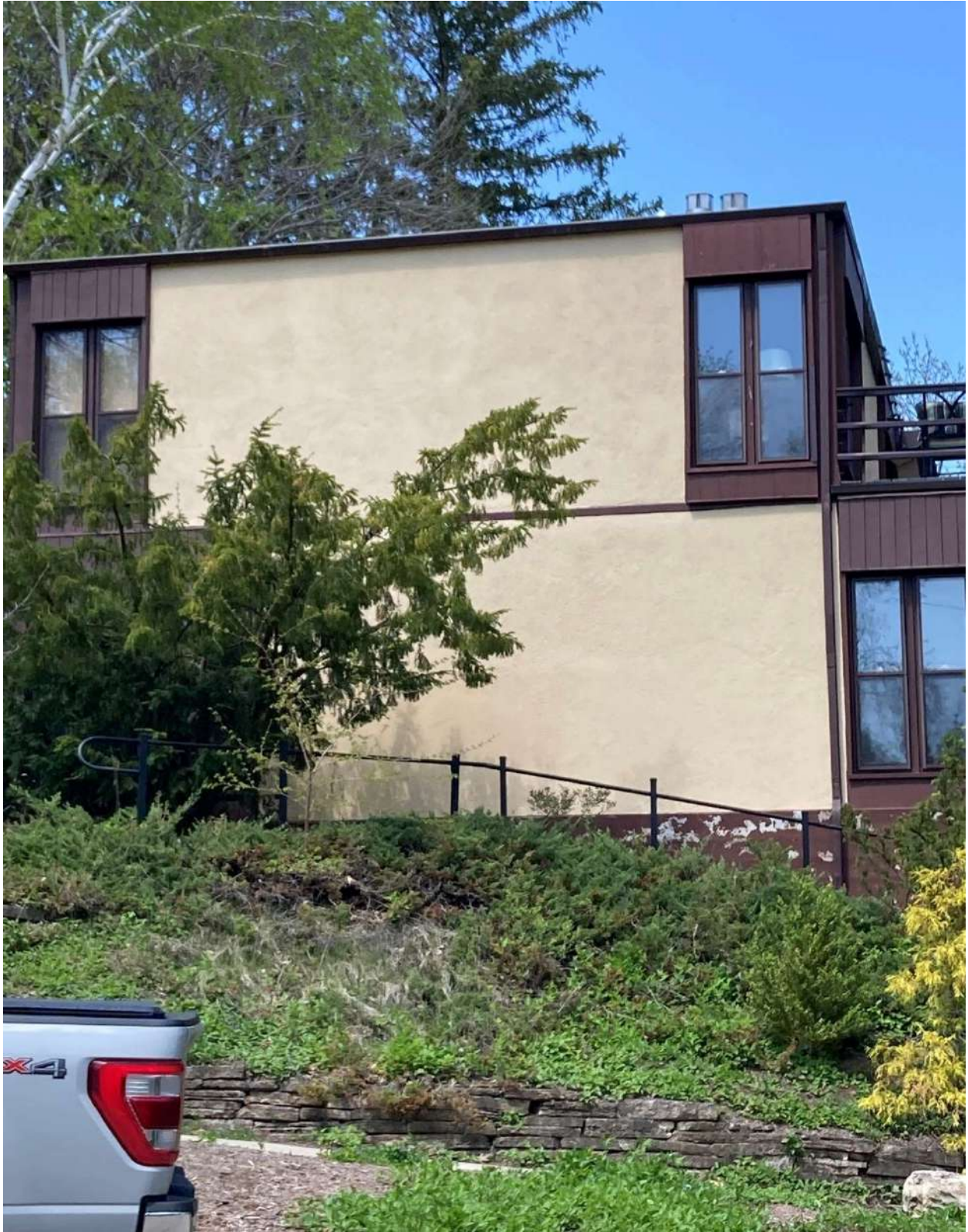
Figure 22 Side view of the Morehouse House, 101 Ely Pl, taken from Summit Ave near the corner with Ely Pl.
