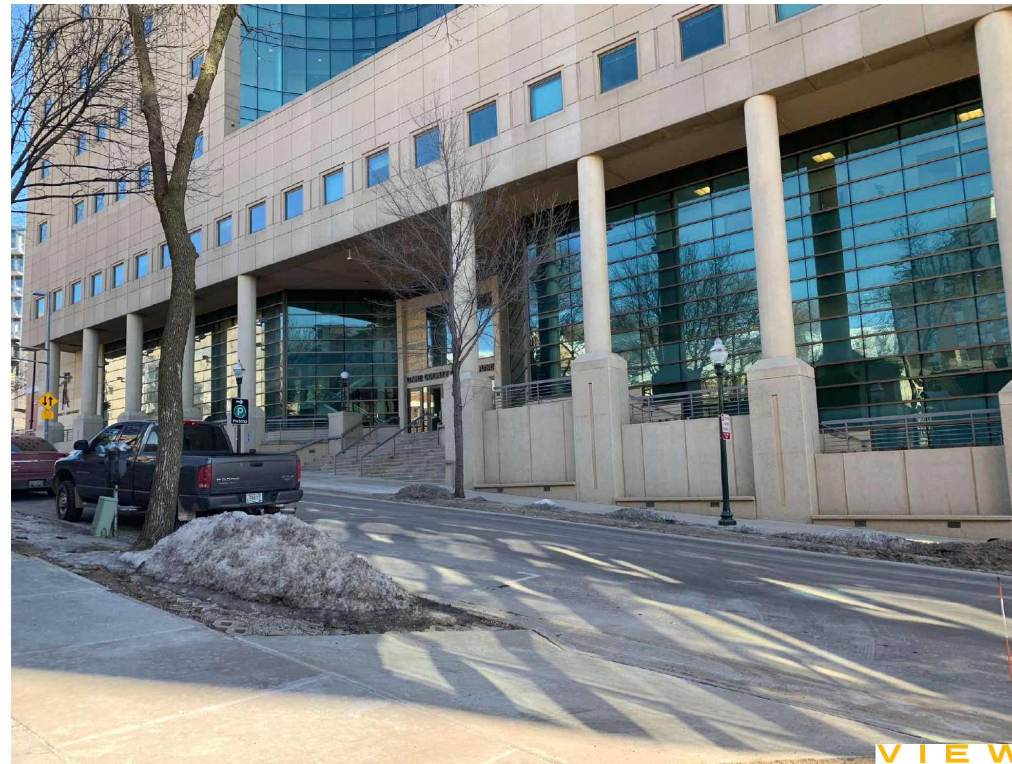
VIEW COURTHOUSE ACROSS HAMILTON
