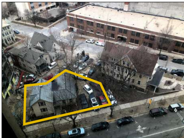
EXISTING SITE FROM S. HAMILTON
