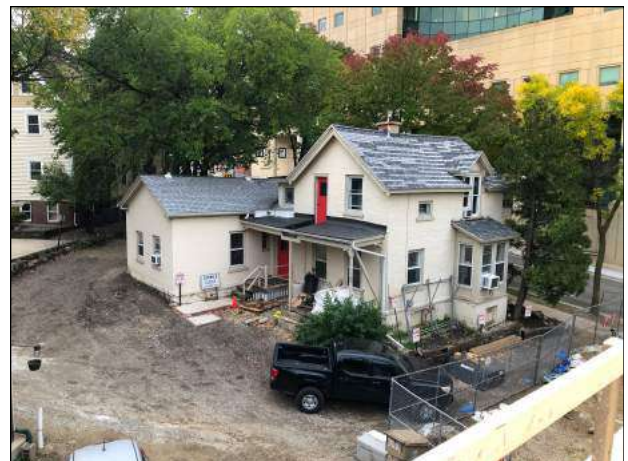
EXISTING BUILDING FROM REAR OF SITE
