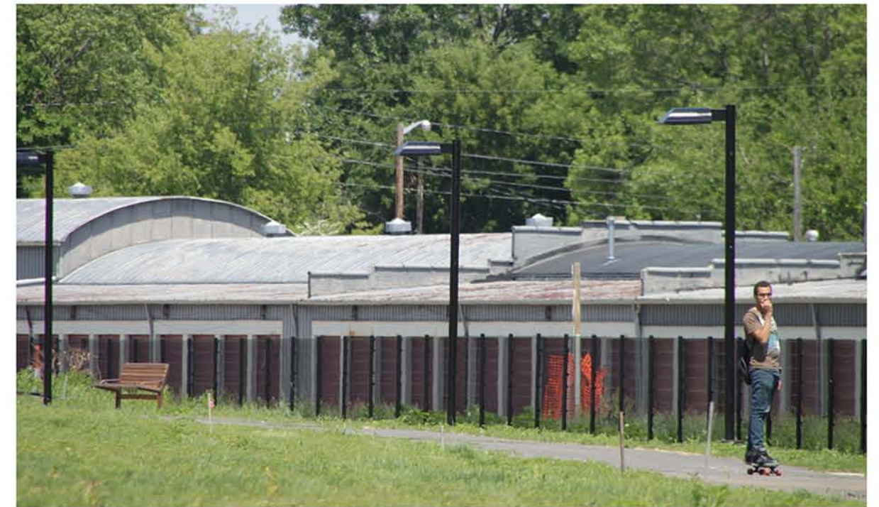
WELDED WIRE FENCE (MATCH CENTRAL PARK)
