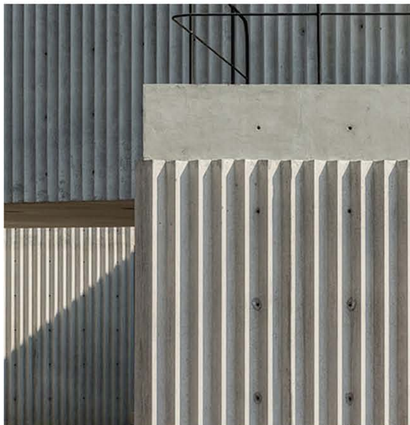
CORRUGATED CONCRETE FORMS housepstudiope.com
