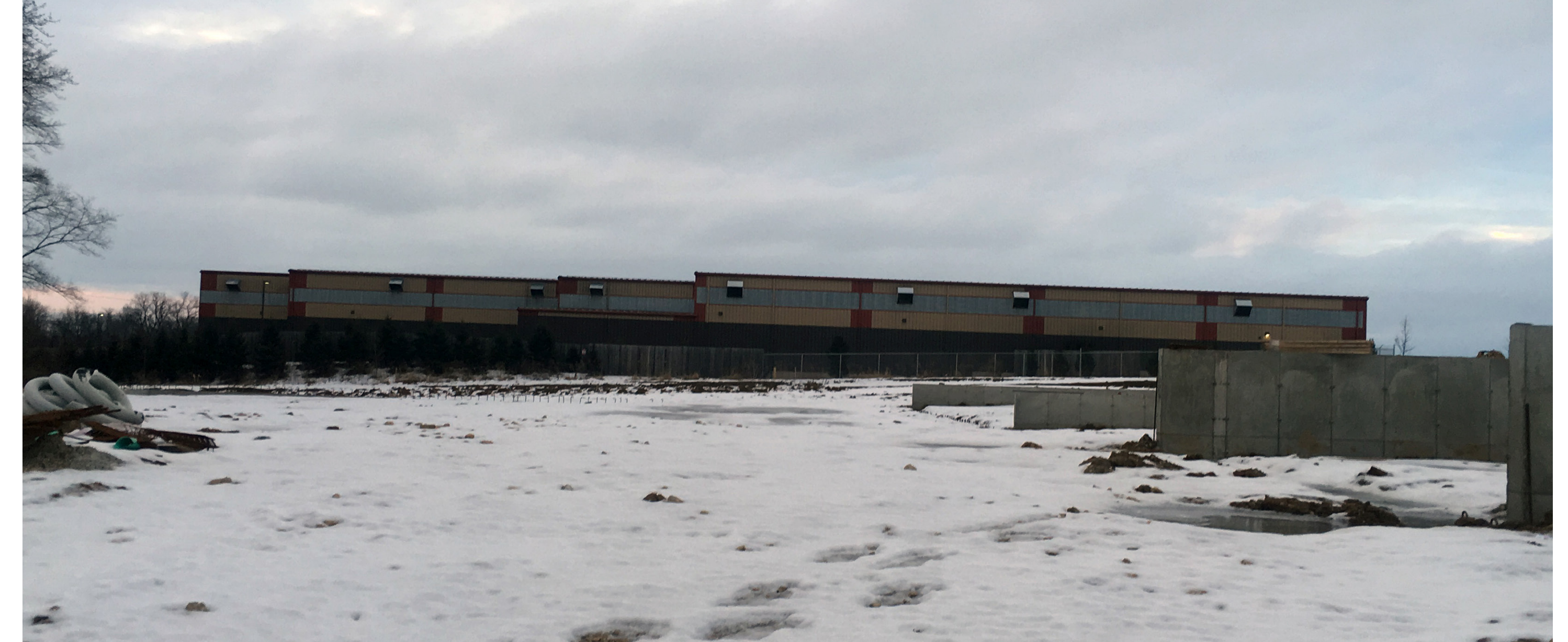
Industrial Building from Marsh Rd.
