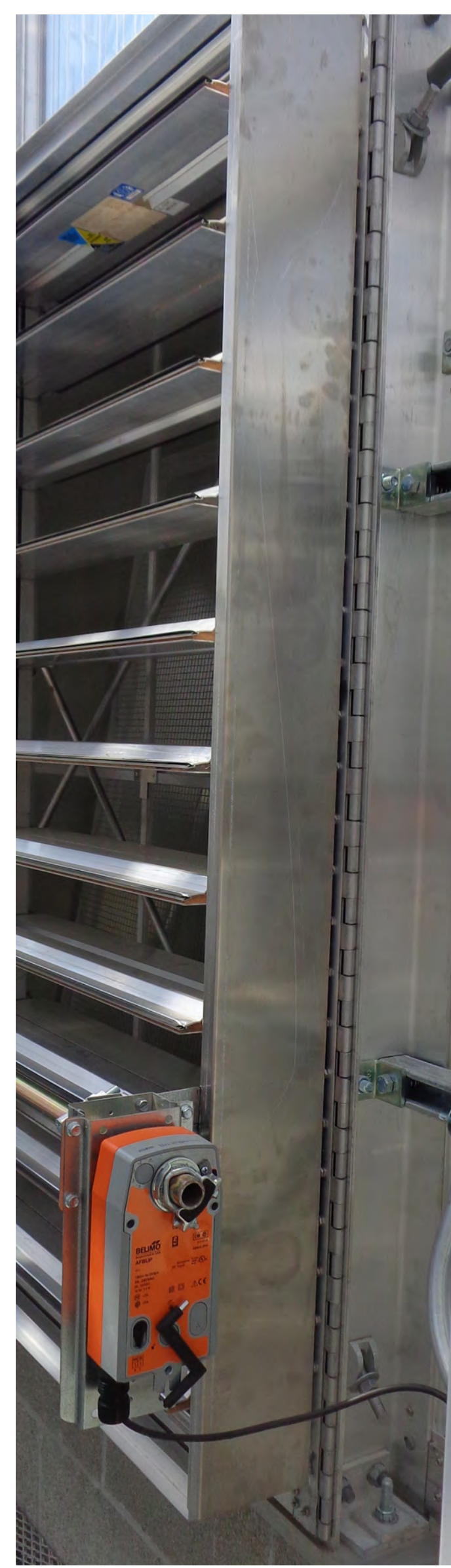
HINGES FOR INSULATED SHUTTERS
