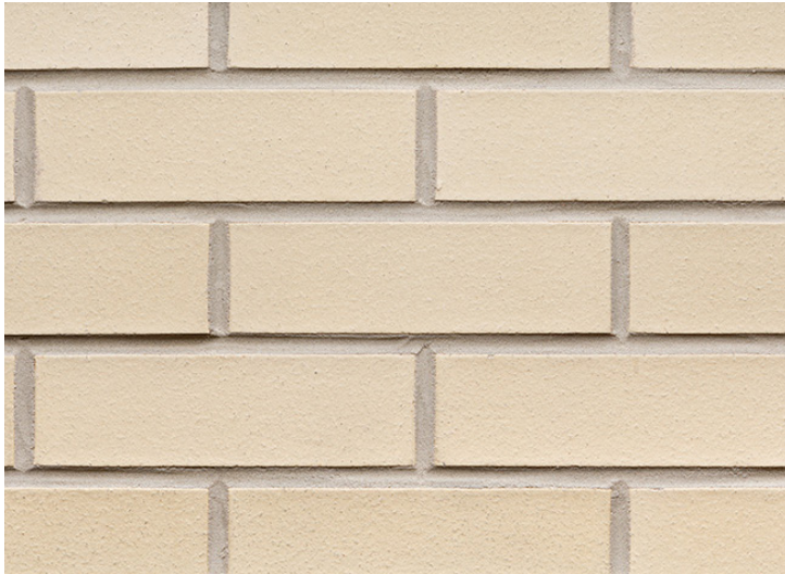
Brick Veneer 2 Cream Brick - 4" x 16" - running
