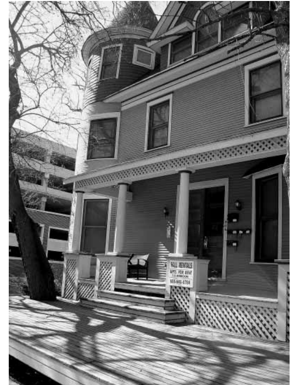
Treated lumber deck detracts from otherwise attractive historic entrance.
