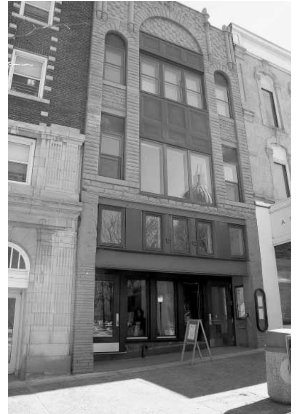
Appropriately restored traditional storefront on N. Pinckney St.
