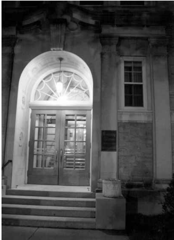
Lighting focuses on entry, does not glare onto adjacent properties and is a warm tone, 1 Langdon St.
