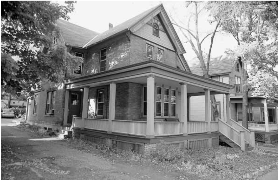
Rehabilitated front porch adding to the interest and character of the home. 110 E. Johnson St.
