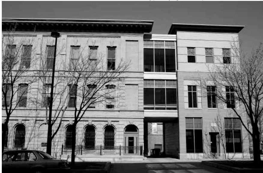
A compatible addition to the American Exchange Bank at N. Pinckney St. and E. Washington Ave.
