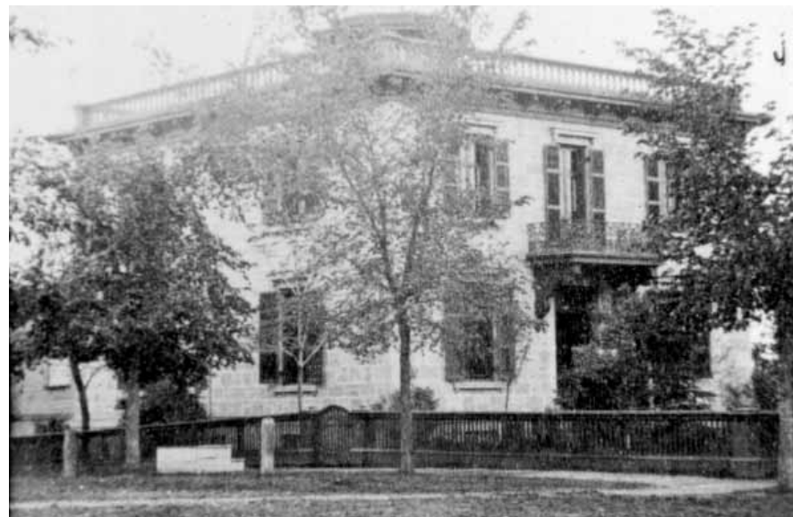
Original Kendall House, 104 E. Gilman St. Built in 1855. Originally styled in the Italianate mode by August Kutzbock with a low-hipped roof and cupola. Wisconsin Historical Society WHI(X3)33389
