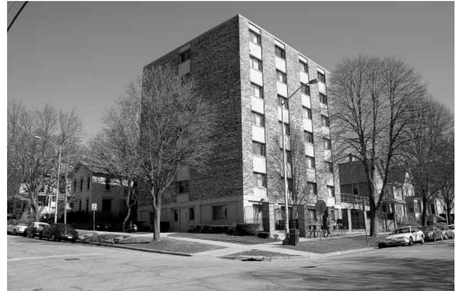
Building which is out of scale with surrounding historic homes.
