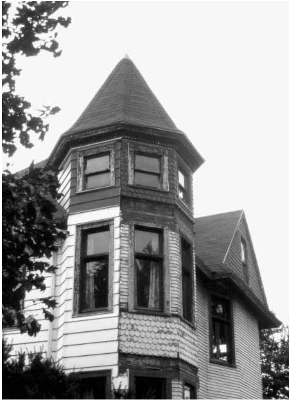
Siding covers important features of the historic home.
