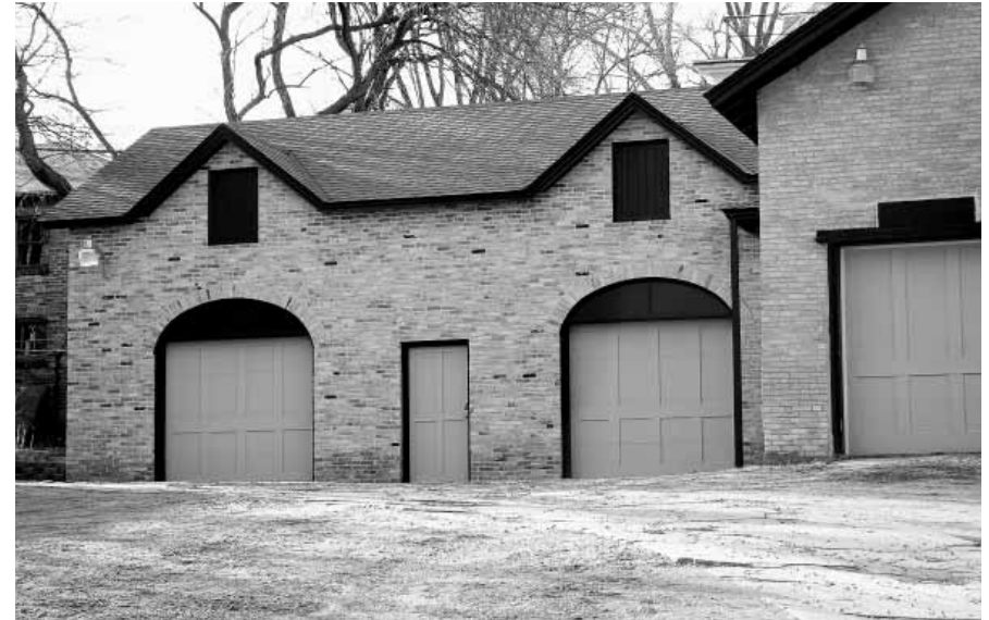
Addition to an outbuilding in the same style as demolished wing using appropriate brick.
