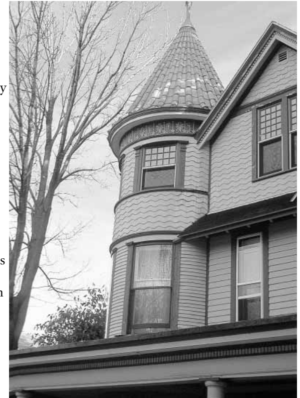
Paint colors appropriately emphasizing architectural details, 125 E. Gilman
