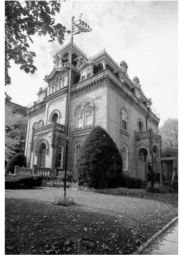
The added mansard roof of the Keenan House at 28 E. Gilman St. has gained historical significance of its own.
