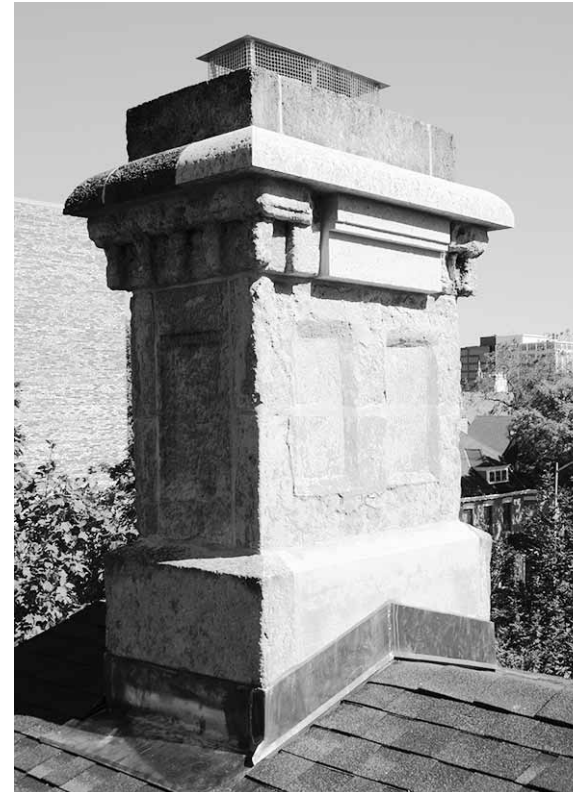
Same chimney as previous illustration which has been rebuilt with the addition removed and the new stone inserted. Dentils yet to be cut.
