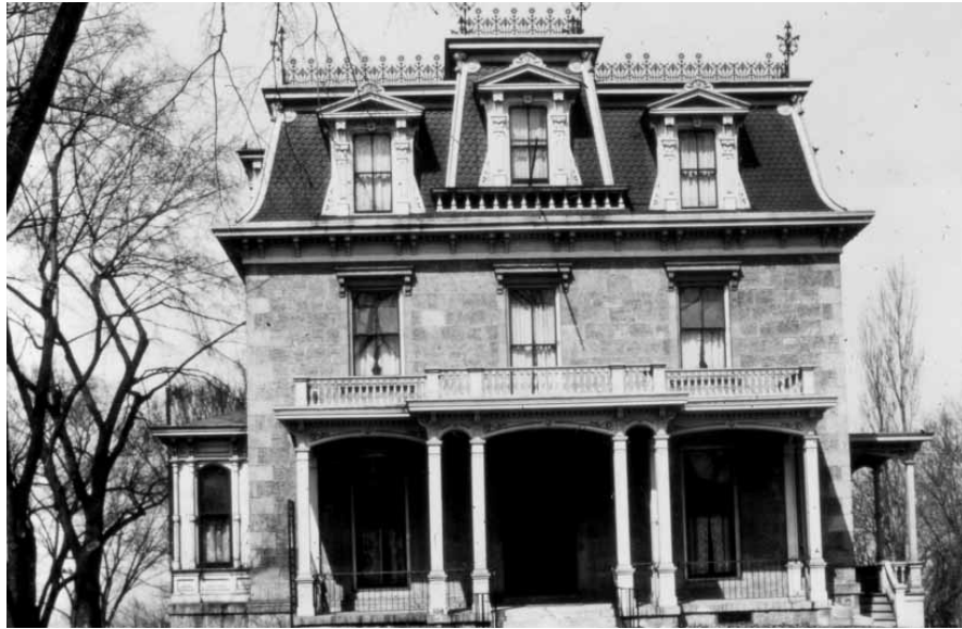
Kendall House 104 E. Gilman St. was restyled in 1873 with a mansard roof to adapt it to the then popular Second Empire style.
