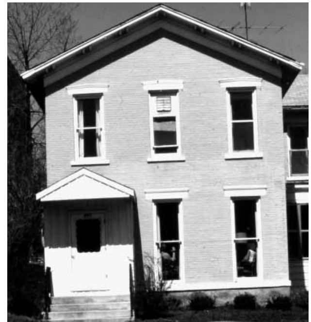
Same house as above with the porch removed diminishing the character and beauty
