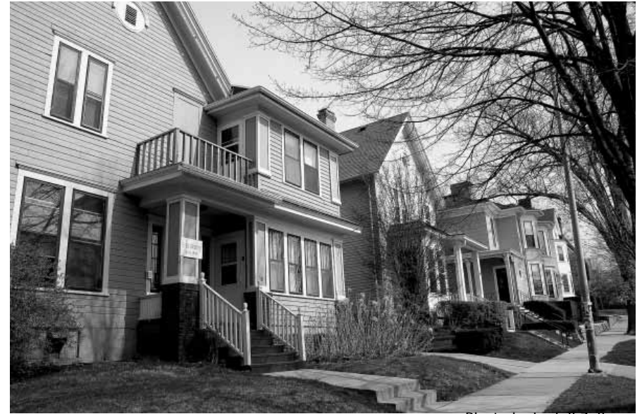
Historic Gilman streetscape showing proportion and rhythm of rooftops and windows.
