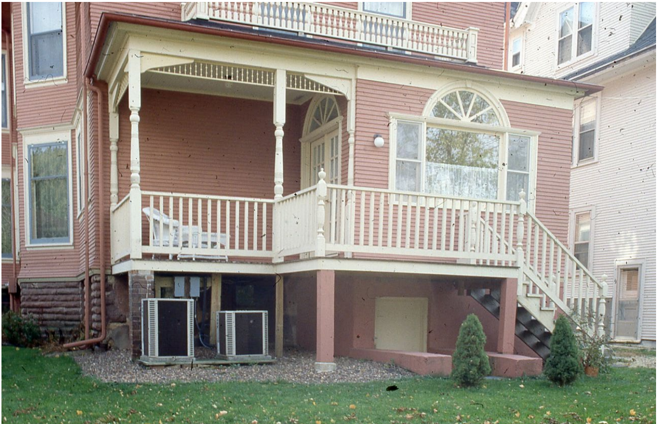
Pre-1980s-remodel photo documentation
