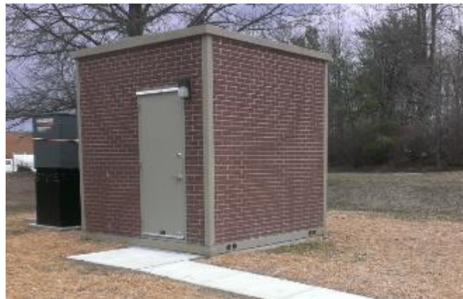
Figure 32: Exterior View – Sample Precast Concrete Shelter with Generator Pad / HVAC
