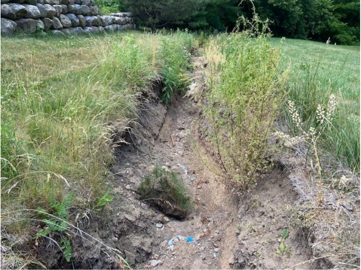
Channel Erosion – Middle Section of Channel
