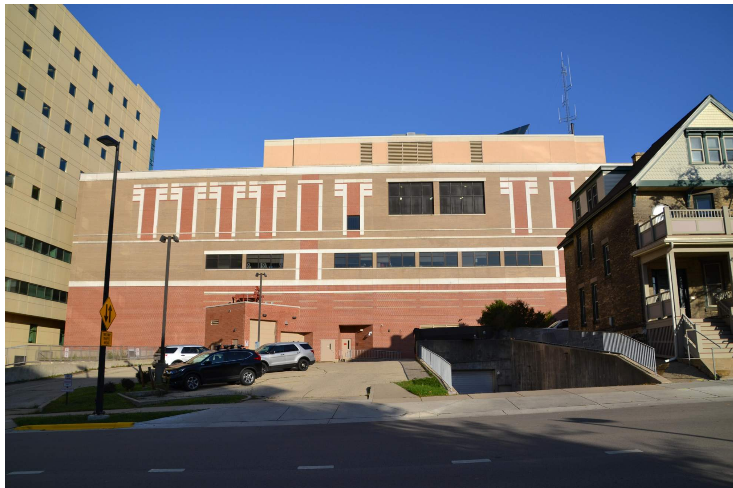
View of Public Safety Building from West Wilson Street
