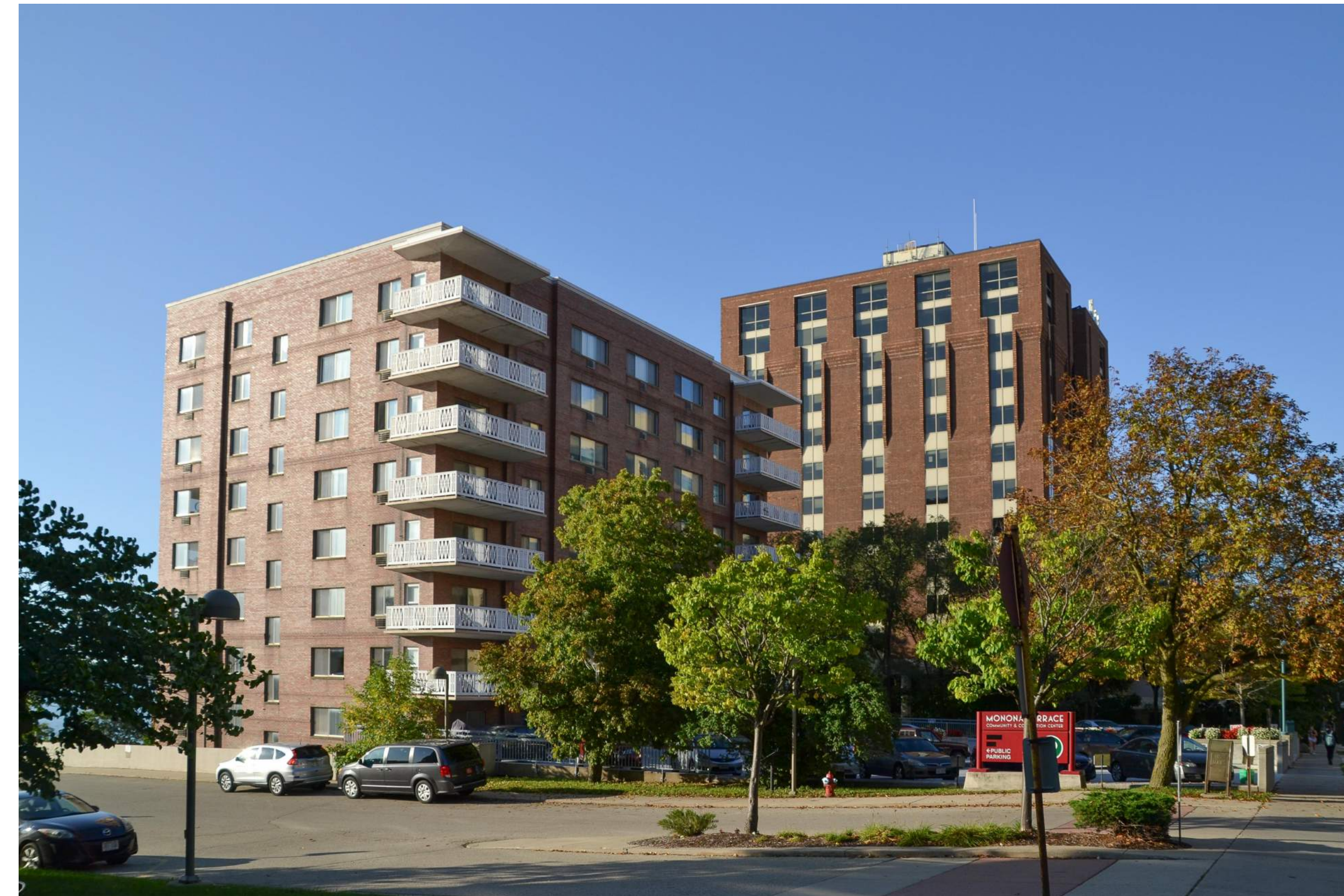
View of 111 West Wilson (Left) and 131 West Wilson (Right)
