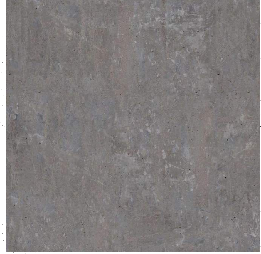
6 CONCRETE COLUMN STAINED, POLISHED
