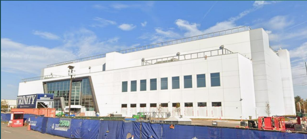
H5 Data Center, Ashburn VA (via Google Street View)
