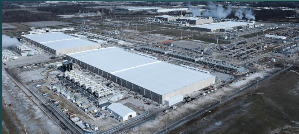
Google Data Center, Council Bluffs IA ( datacenters.google )
