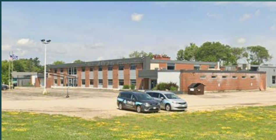
Data Center, 4916 East Broadway, Madison WI
