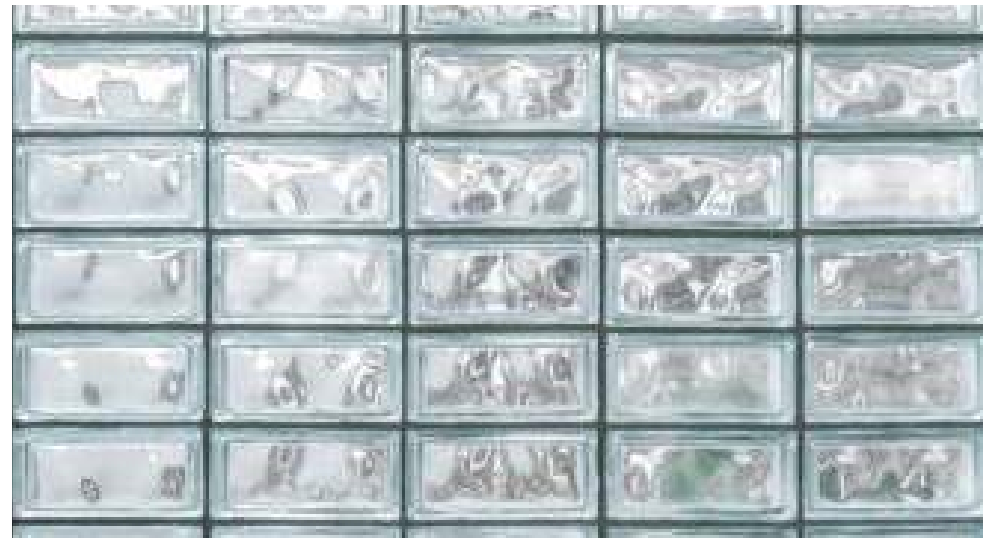
GLASS BLOCK - CLERESTORY WINDOWS AT BASE
