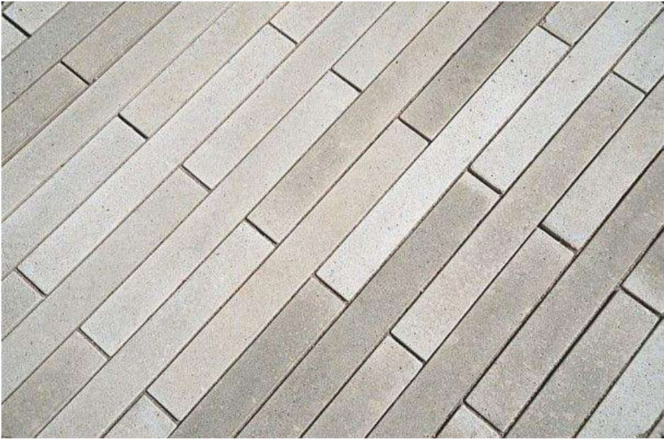
WALKING SURFACE SMALL SCALE RUNNING BOND PATTERN
