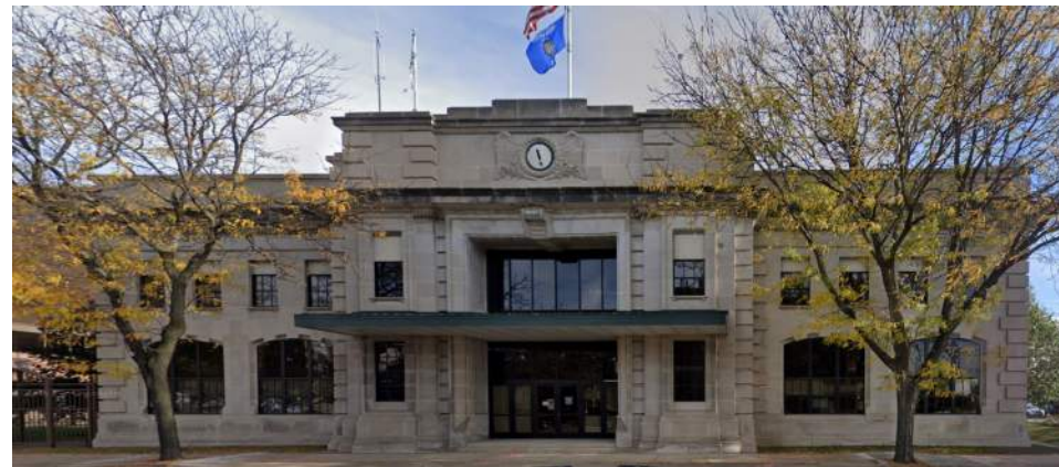
631 RAILROAD ST. FLAT ROOF, MASONRY, DOUBLE-HEIGHT ENTRY EXPRESSION, BASE WAINSCOT, CORNICE EXPRESSION, WINDOW GROUPINGS, RELATIVE SCALE, BEAUX ARTS STYLE, ARCHED WINDOWS
