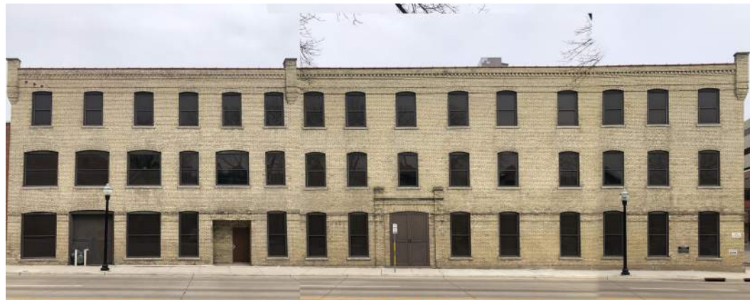
602 RAILROAD ST. FLAT ROOF, MASONRY, WINDOW PROPORTIONS, CORNICE EXPRESSION, RELATIVE SCALE, ARCHED WINDOWS
