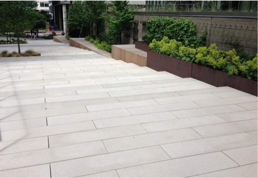
DRIVE ISLE LARGE SCALE RUNNING BOND PATTERN
