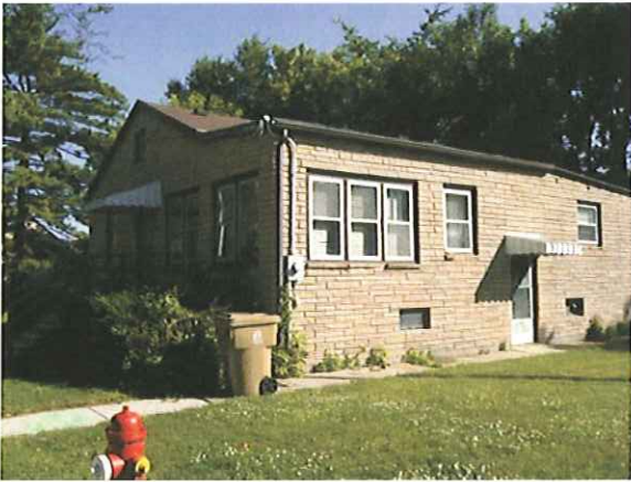
Photo of existing home at 171 Proudfit Street
