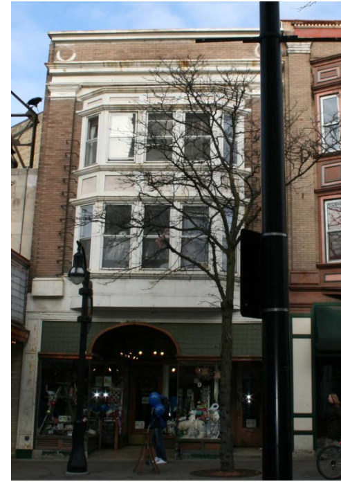
Schumacher Building (214 State Street)
