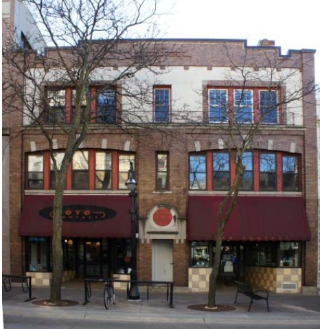
121-123 State Street, C.E. Buell Building State and Fairchild Street construction
