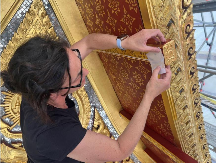
*Figure 2: A contractor from Kalam applies new gold leaf to areas where it has worn off.*
