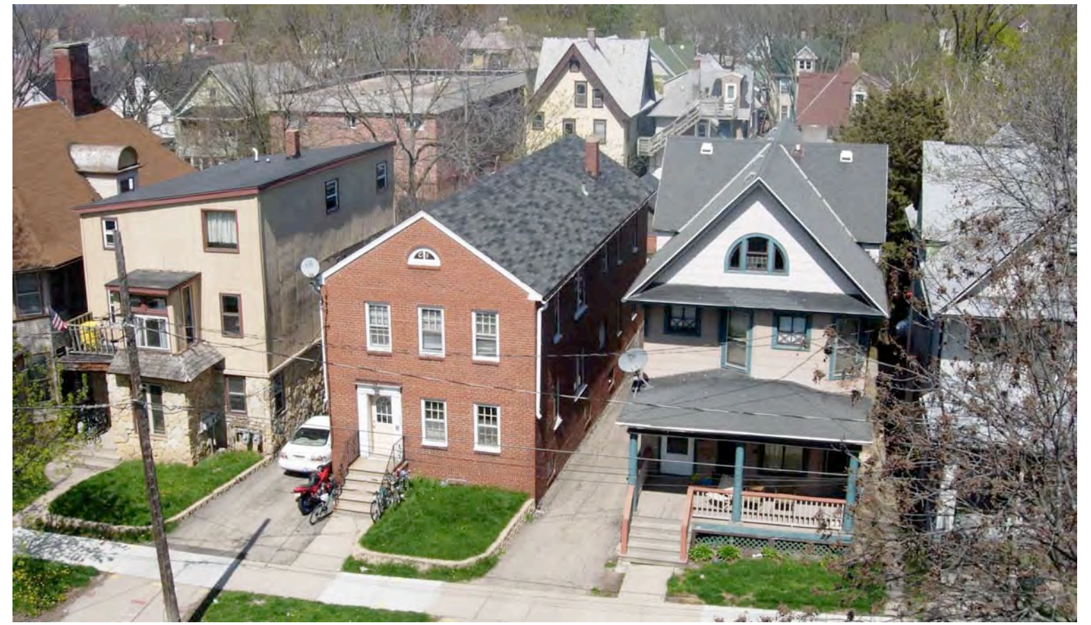
View from the South West of 119, 123 & 125 North Butler
