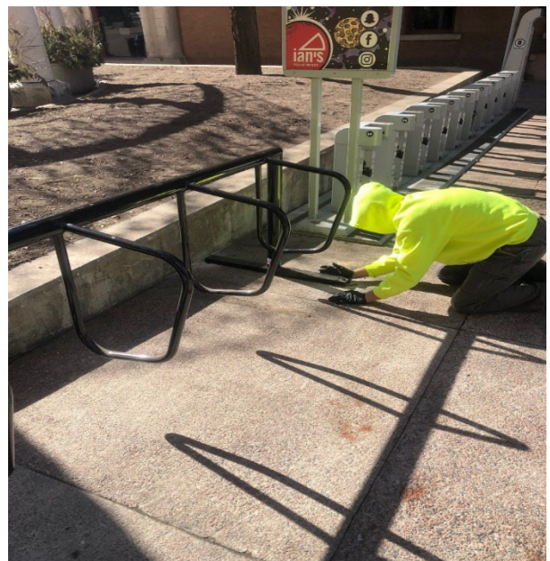
Bike rack installation
