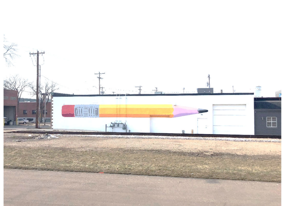
ADDITION ON TOP OF BUILDING
