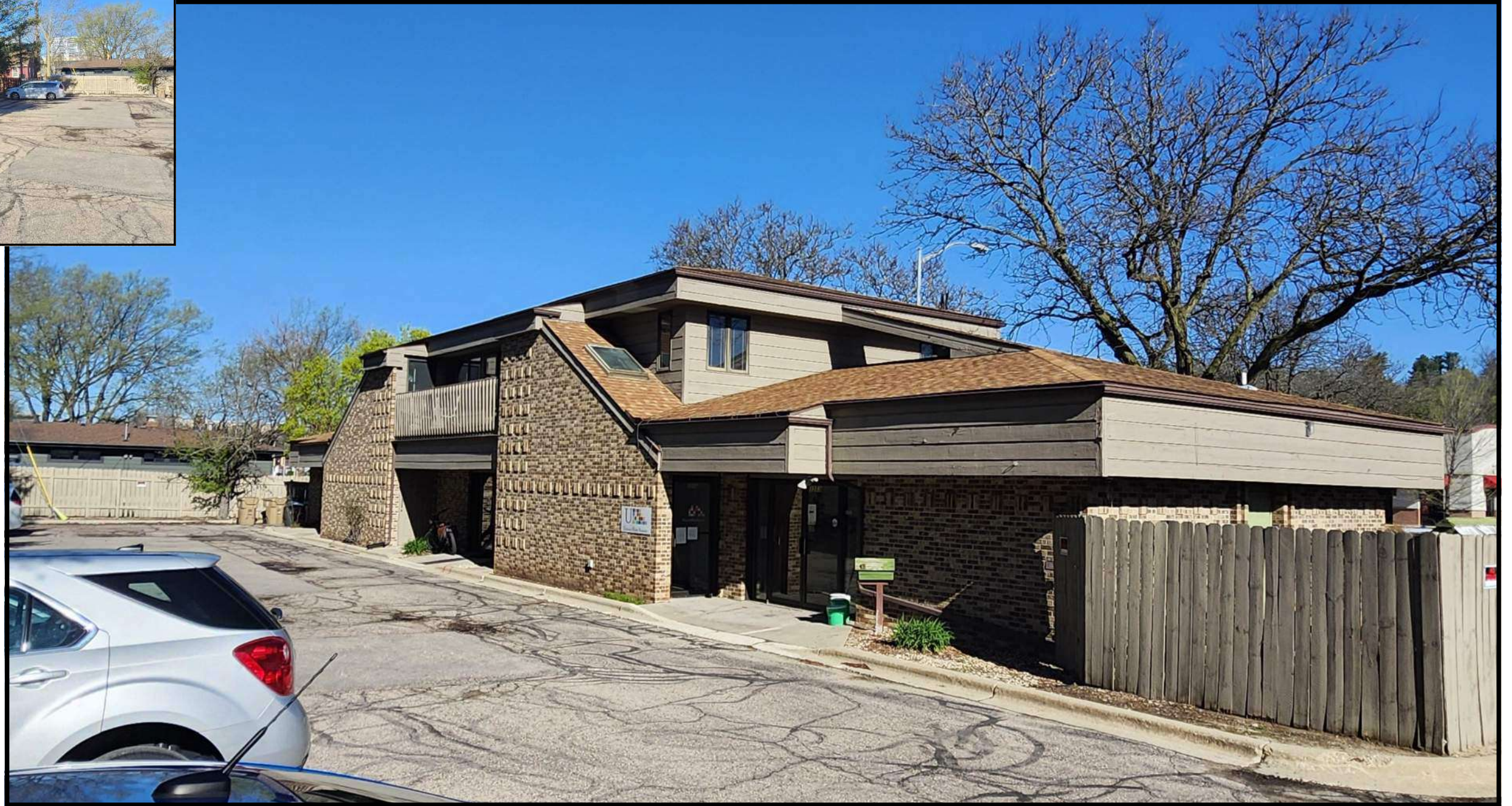
WEST BUILDING - REAR
