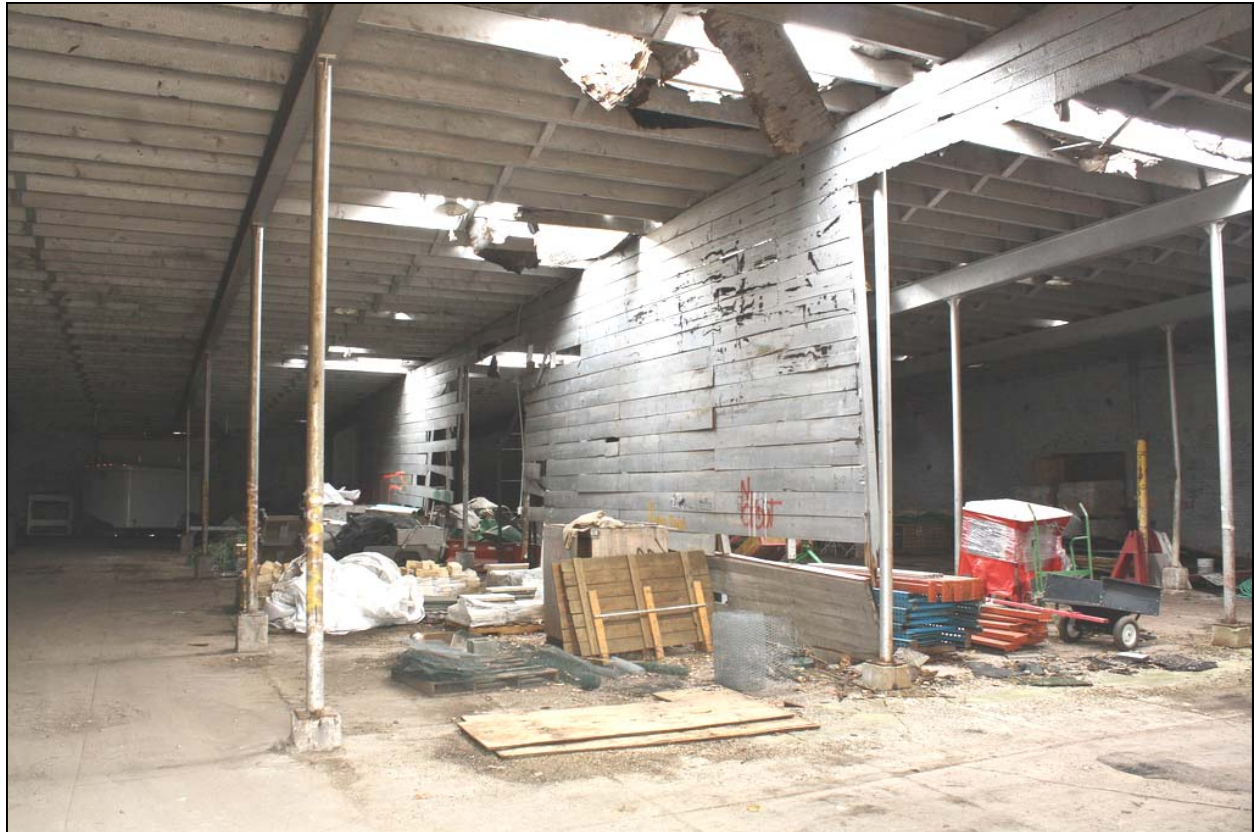
Image 32: Interior of former storage building.
