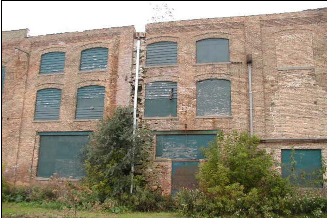
Image 16: North elevation detail.
