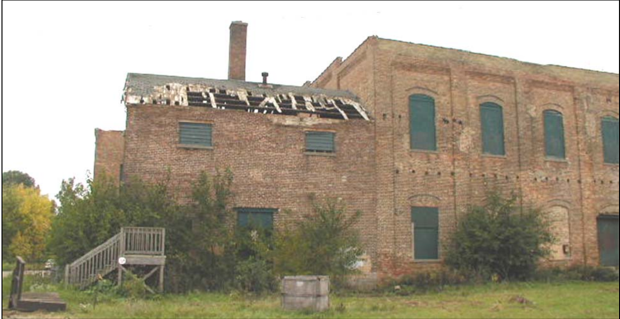
Image 14: North elevation, looking south.
