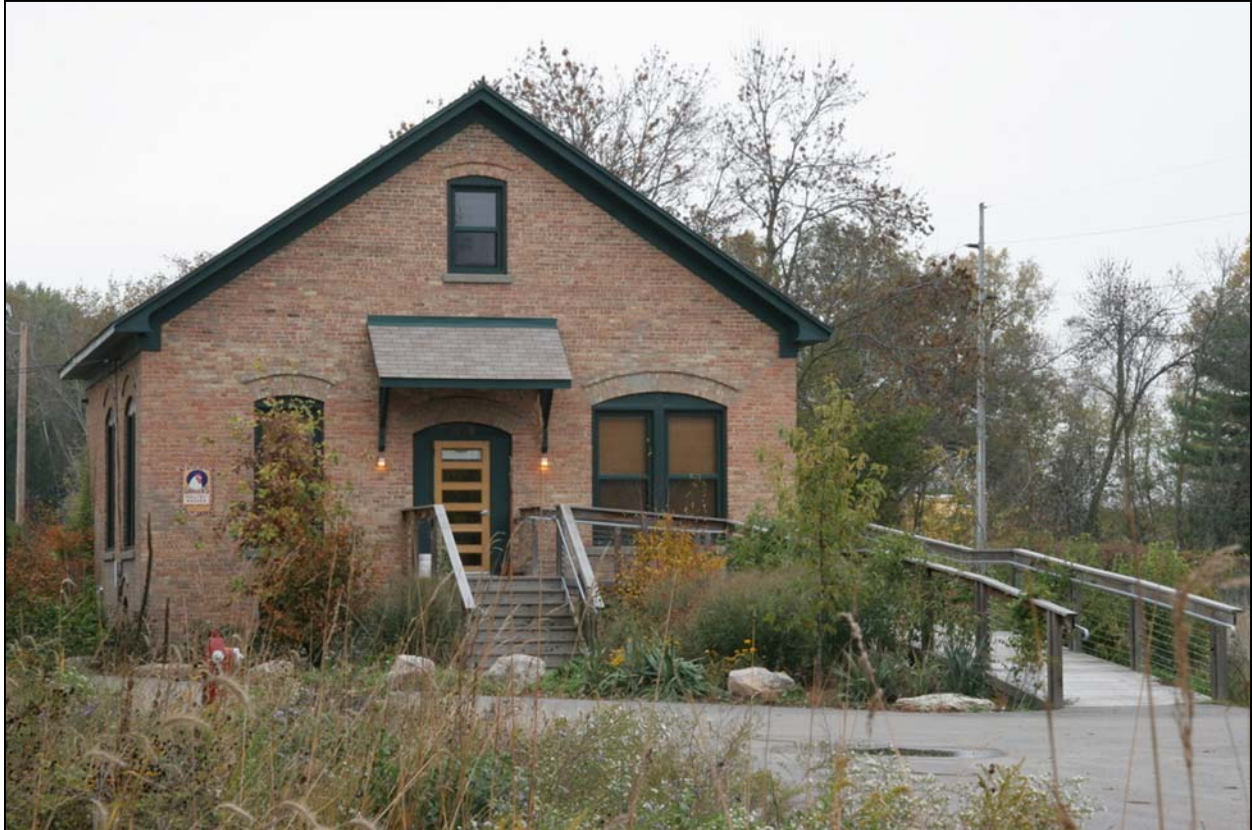
Image 24: West elevation of office building.
