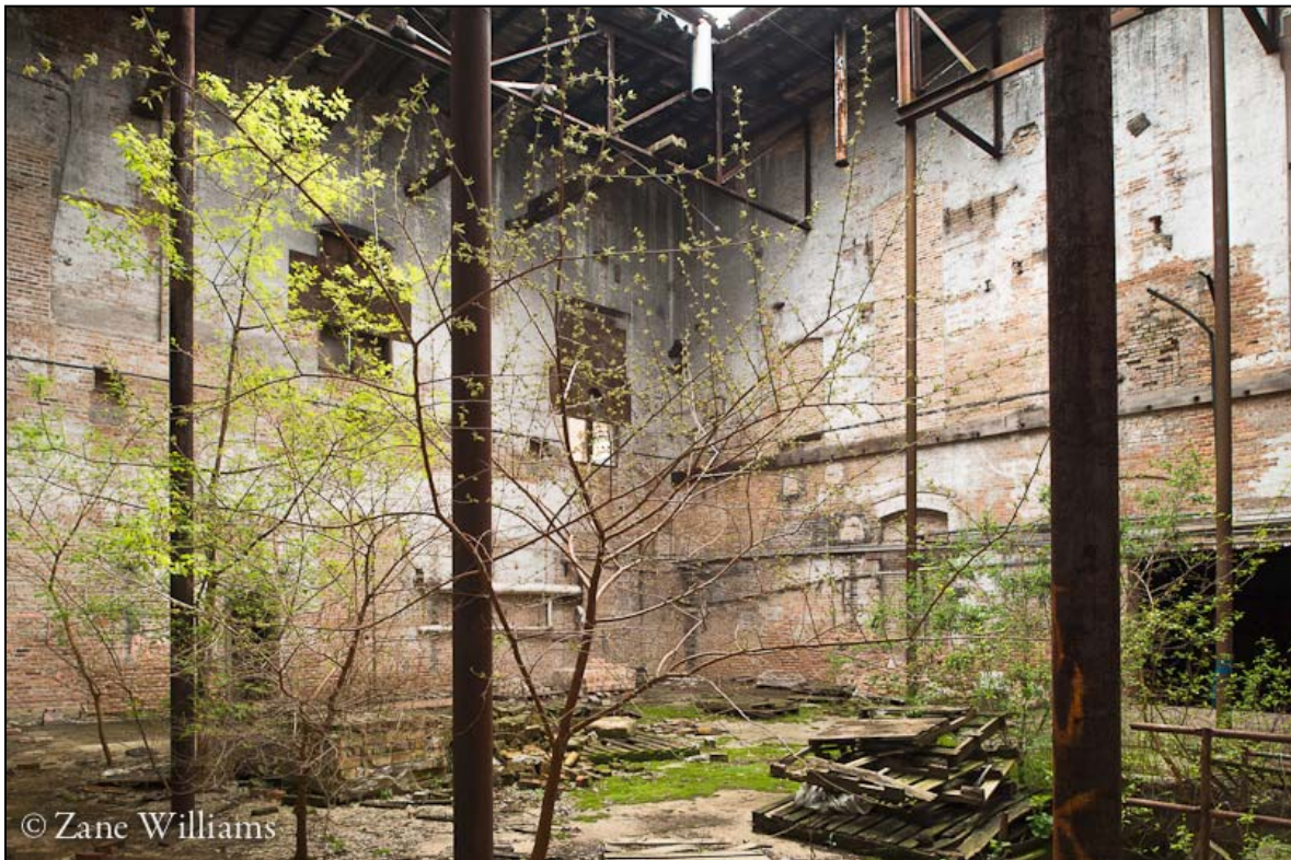
Image 29: Interior of former feed storage area.
