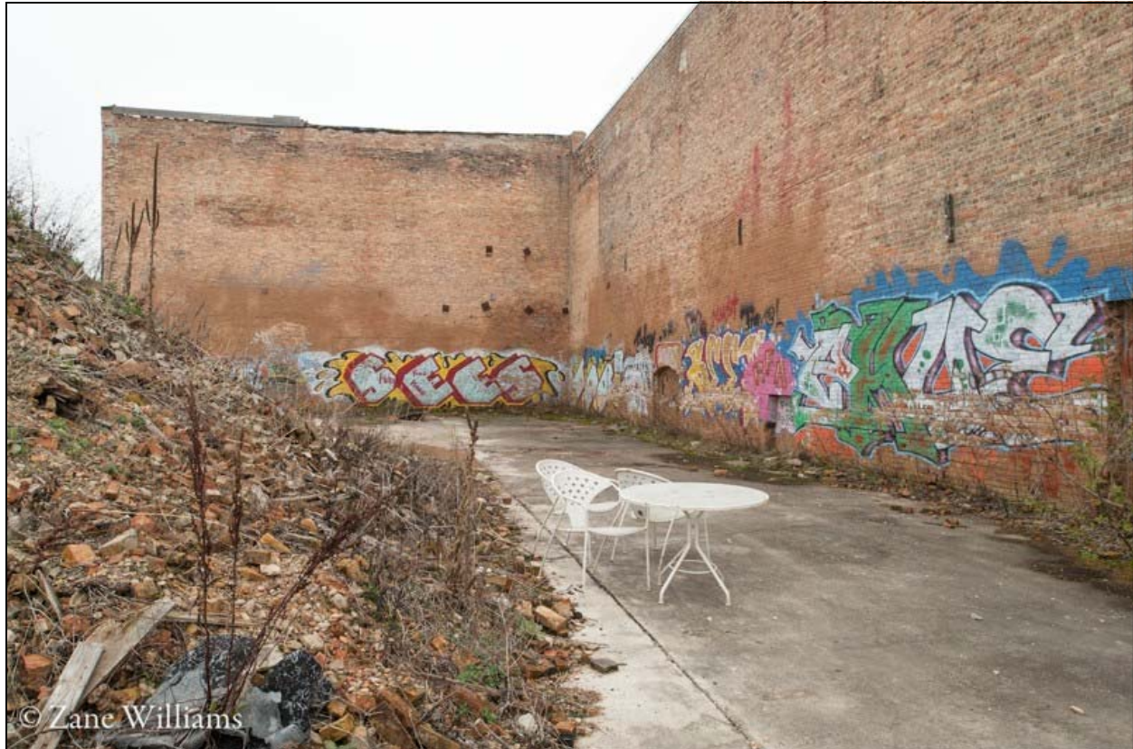
Image 18: North elevation, looking east.
