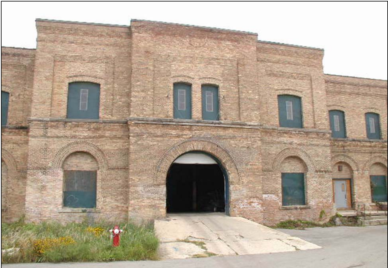
Image 11: South elevation, entrance detail.
