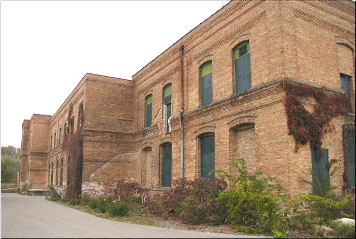
Image 12: South and east elevations, looking northwest.
