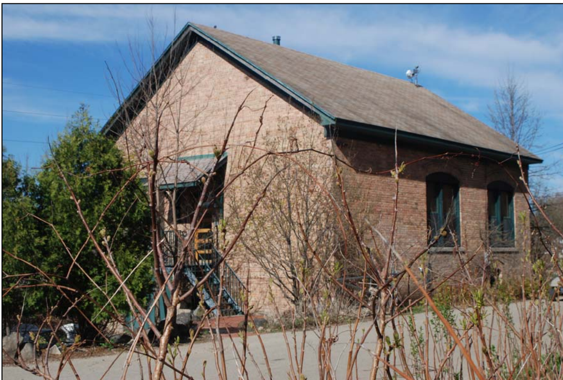
Image 25: West and south elevations of office building.
