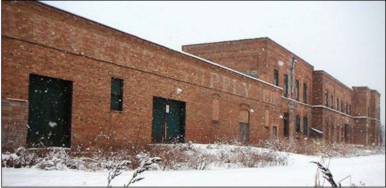
Image 22: South elevation, looking northeast.
