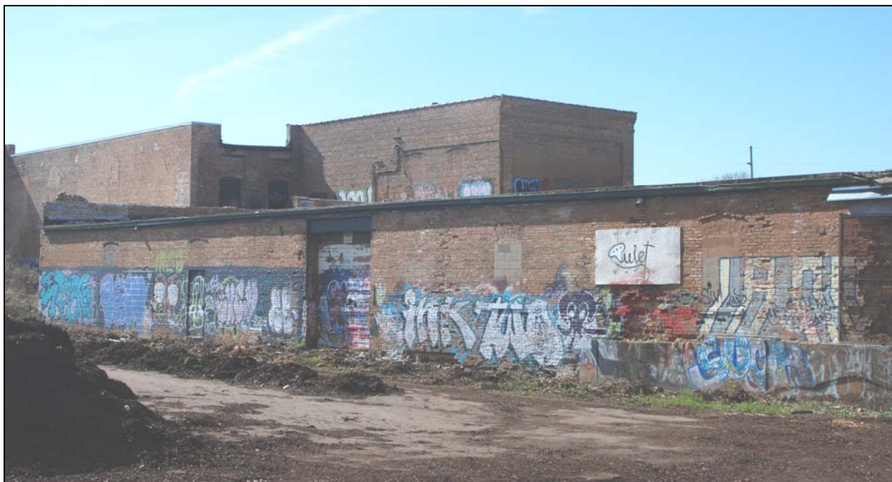
Image 19: North elevation, looking southeast.
