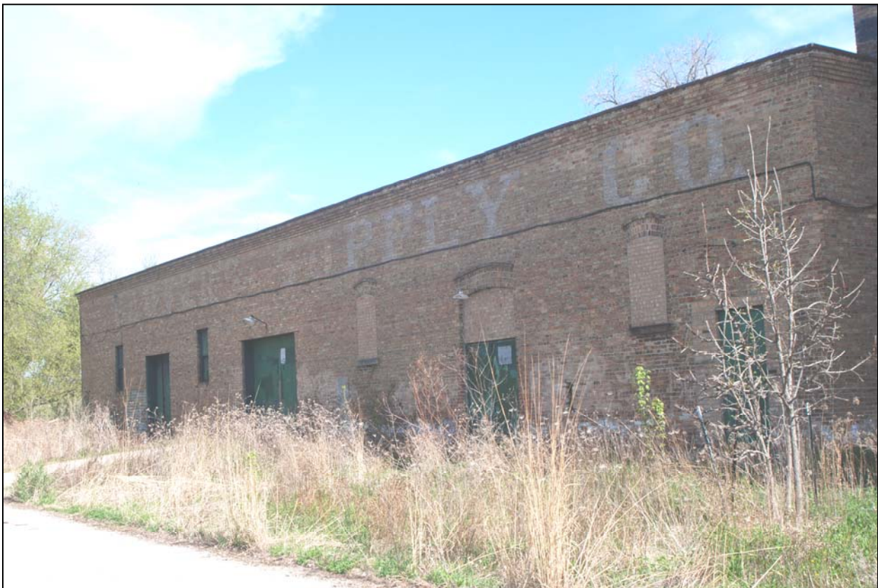
Image 21: south elevation of storage building, looking northwest.
