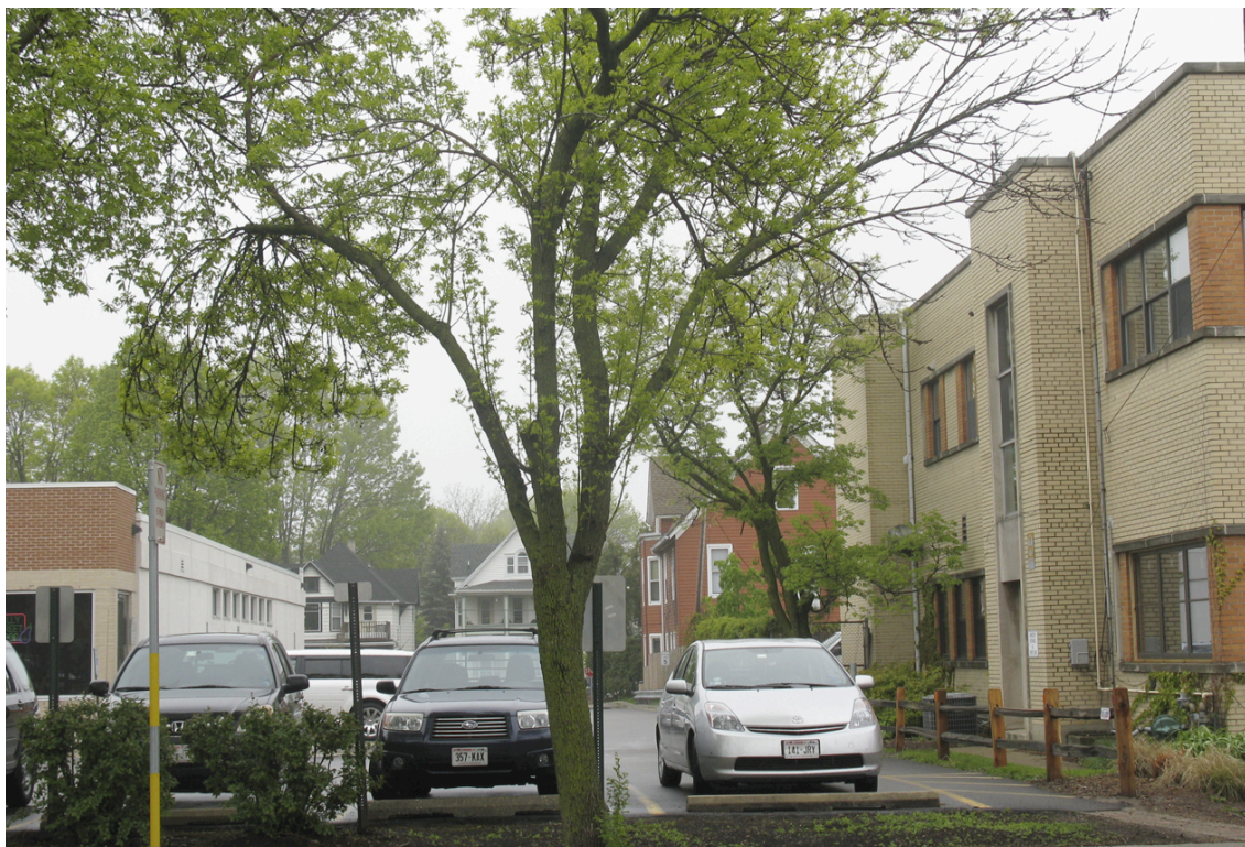
WEST WALL AND PARKING LOT OF COOPERATIVE LOOKING SOUTH ACROSS WILLIAMSON STREET
