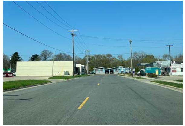
Roth Street (cracking, curb crumbling)
