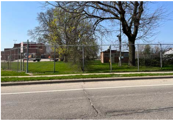
Aberg Avenue (cracking, crumbling, settling)
