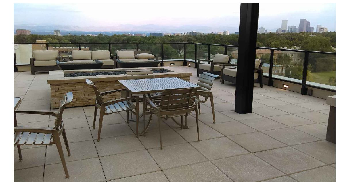
COURTYARD PAVER: 2'X2' CONCRETE PAVER ON PEDESTAL SUPPORT SYSTEM, COLOR TO BE DETERMINED
