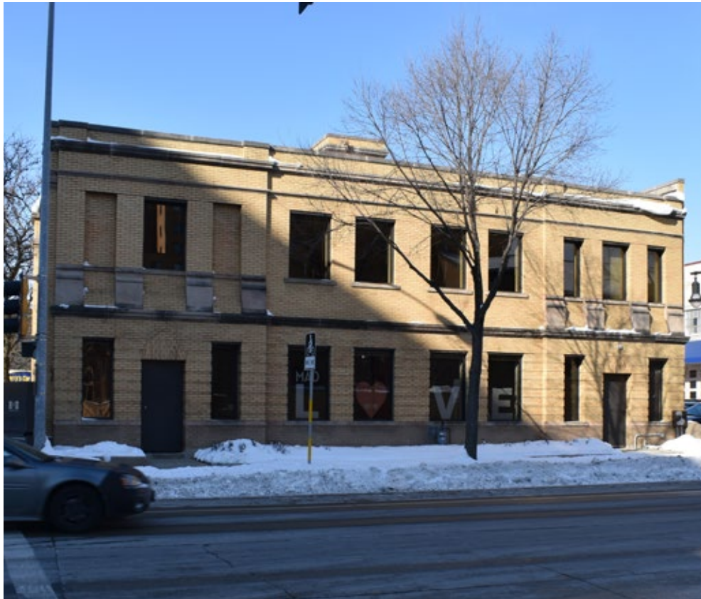
301 W JOHNSON STREET
