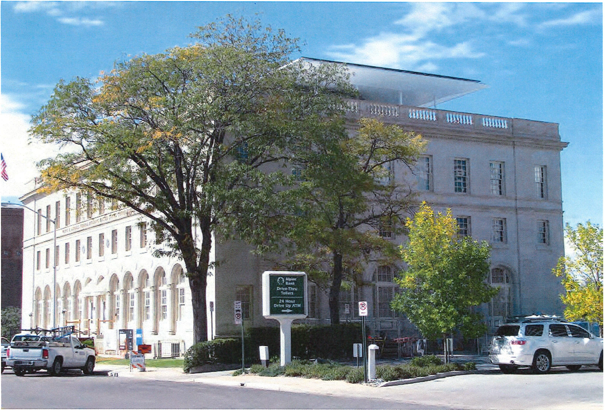
Aspinal Federal Building
