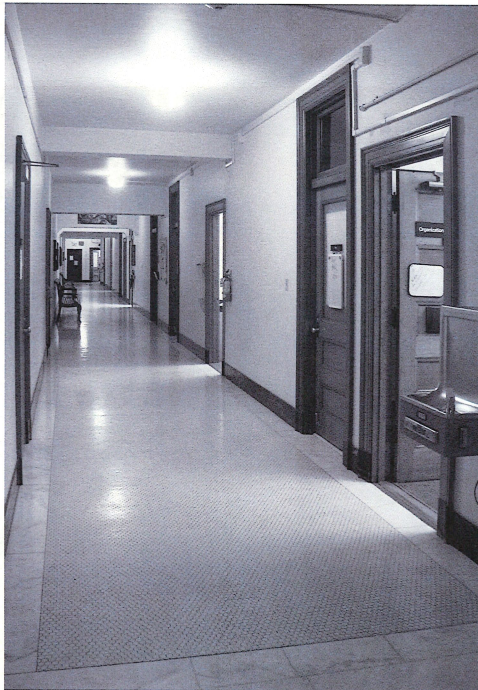
Upper Floor Corridors
