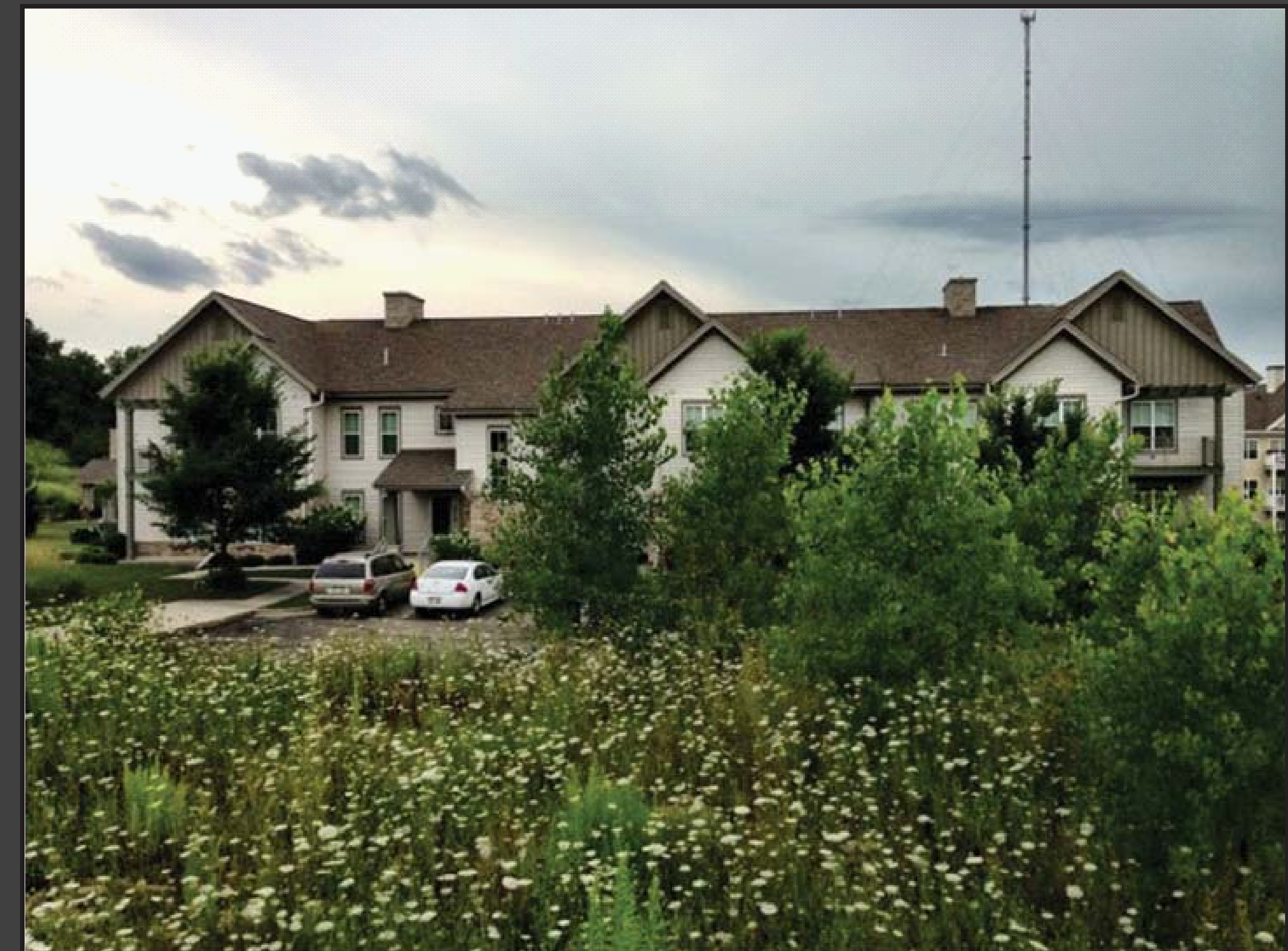
12 UNIT CONDEO, HILLSIDE ESTATES
