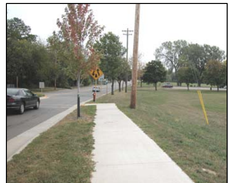
The recent removal of the West Olin Avenue bridge has opened up access to Franklin Field. Sidewalks should be extended along the northern side of Franklin Field.
