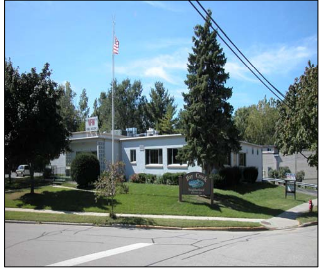
The VFW club is located at a key corner and provides vital functions for veterans. This premier site has the potential to be redeveloped at a higher density than today.
