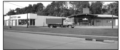
The vacant gas station and tire store site at South Park Street and West Badger Street redevelopment project.
