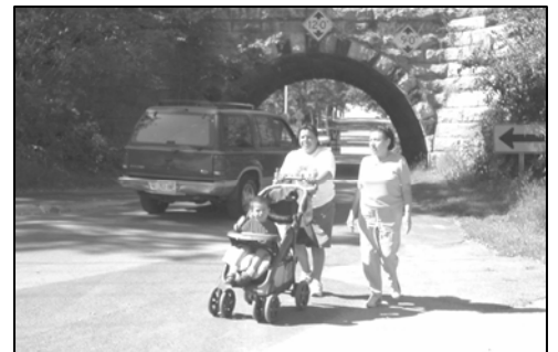
Access to Quann Park from the Bram's Addition Neighborhood is unsafe since pedestrians must walk through a narrow railroad viaduct.
