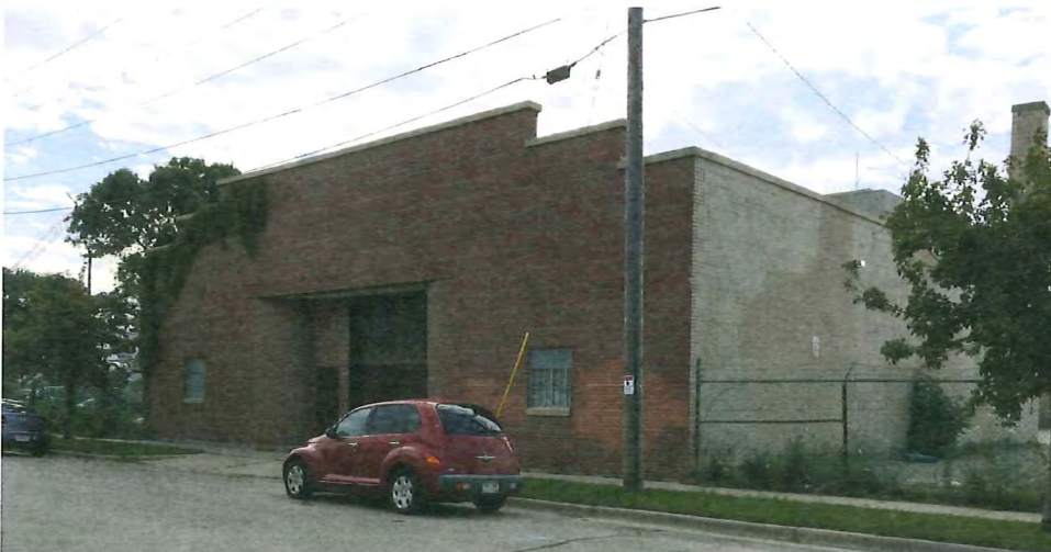
To be Demolished - 910 East Main Street
