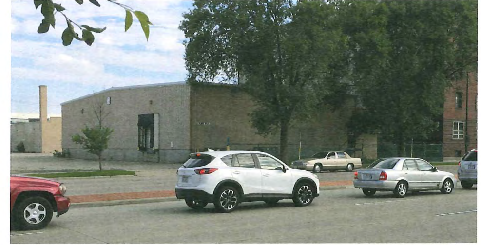
To be Demolished - 905 East Washington Ave.
