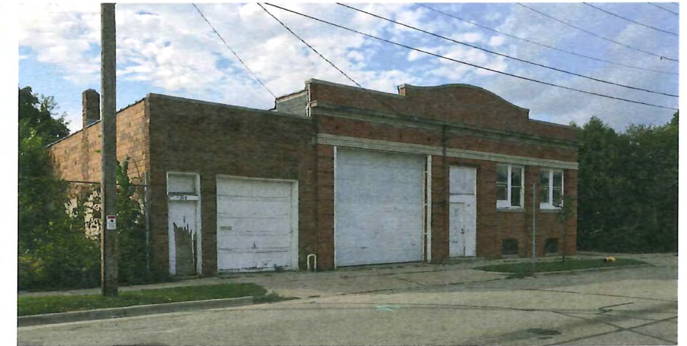
To be Demolished - 922, 924 East Main Street
