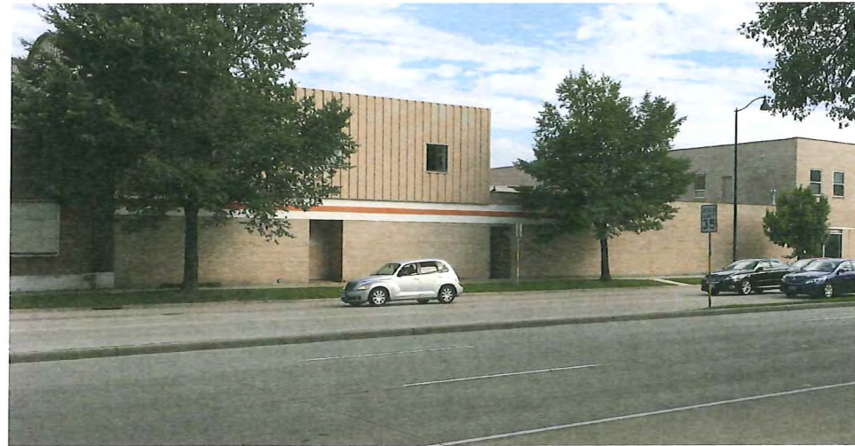
To be Demolished - 939 East Washington Ave.
