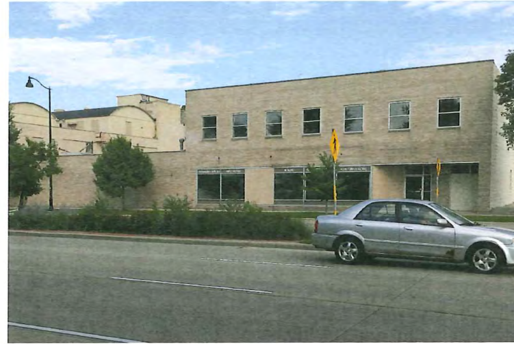
To be Demolished - 925 East Washington Ave.
