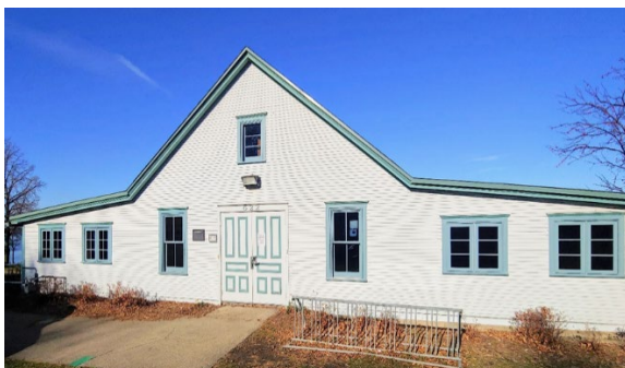
Hoover's Boat House window replacement
