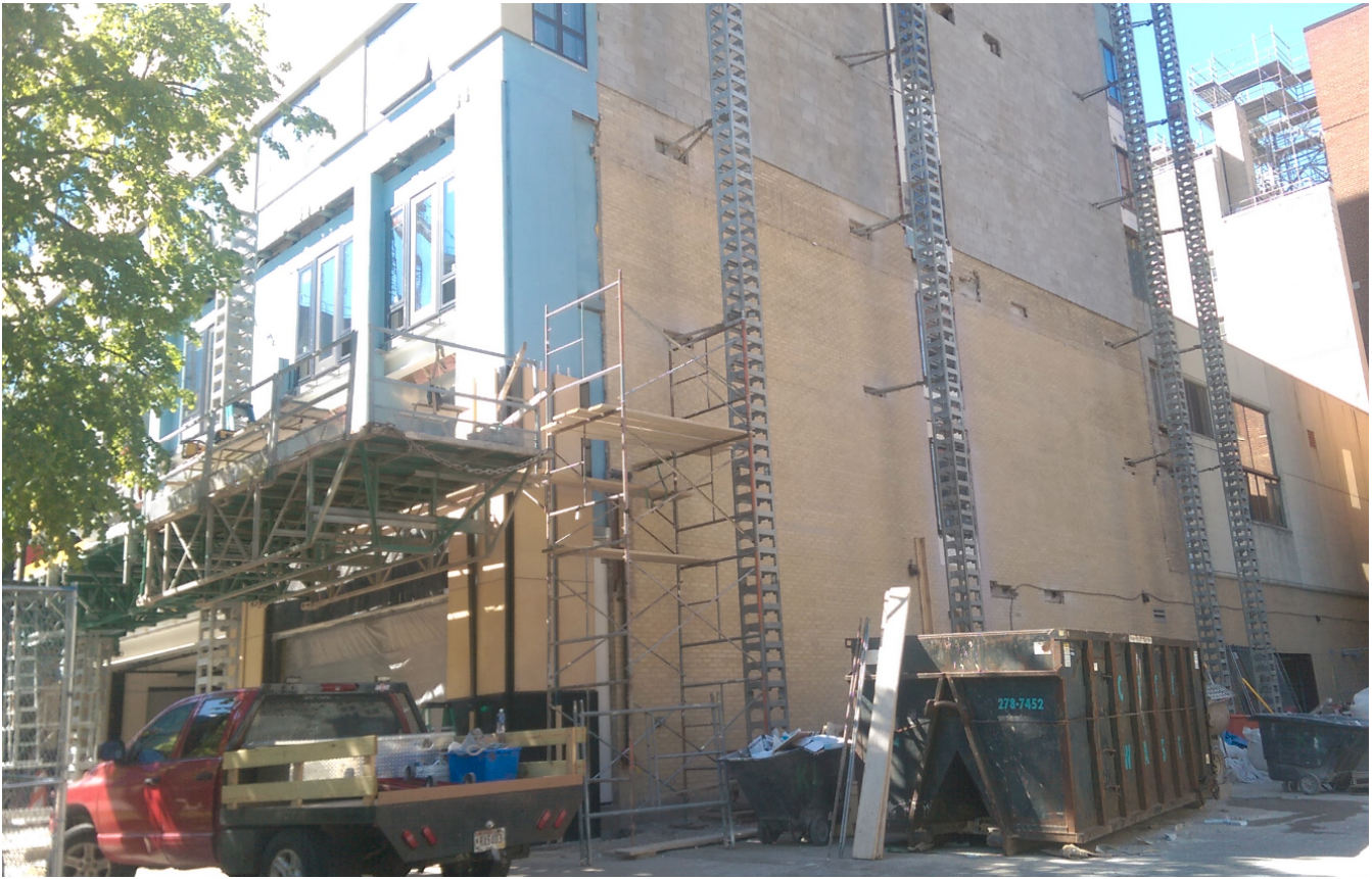
North Elevation – May 18, 2016
