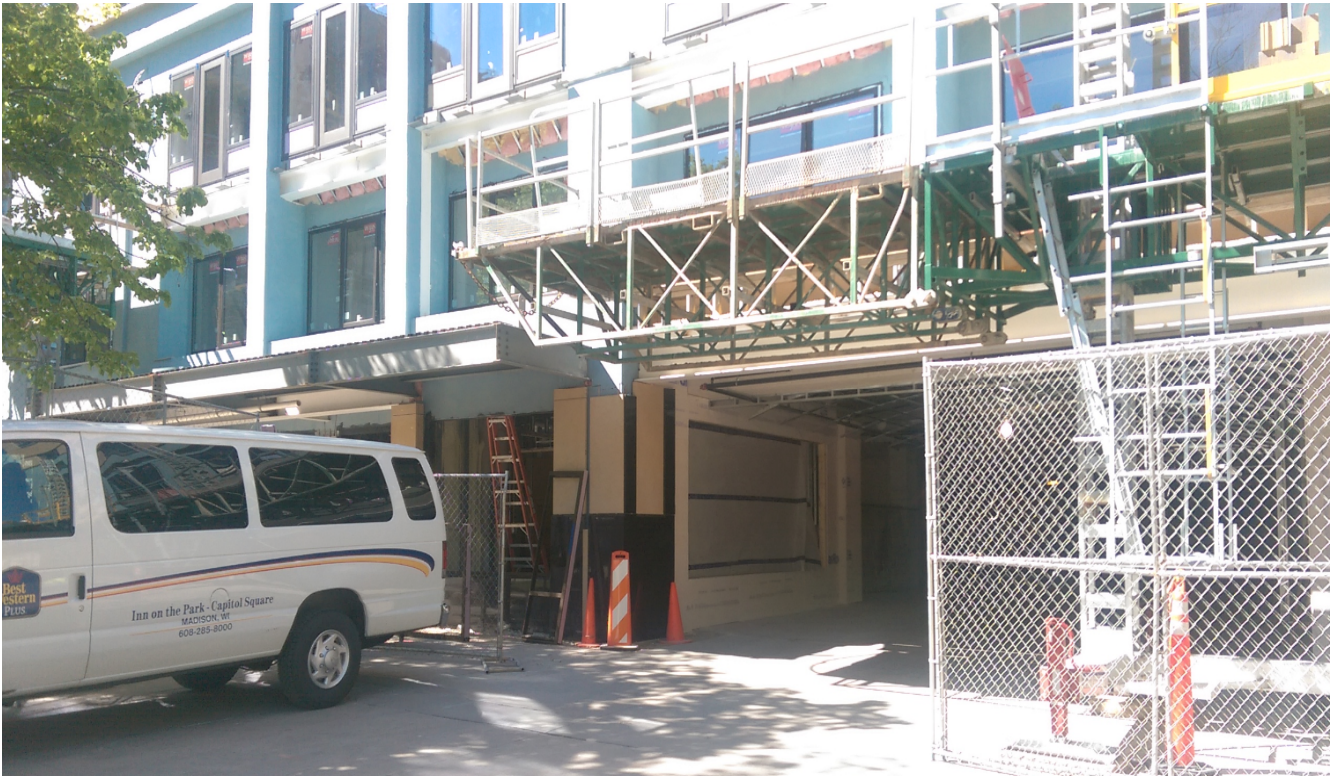
Carroll St – Marquee framing and Valet Entry
