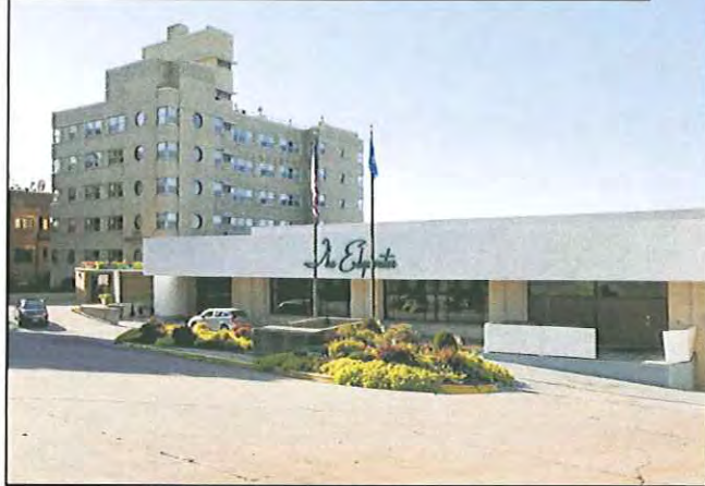
EXISTING EDGEWATER HOTEL
