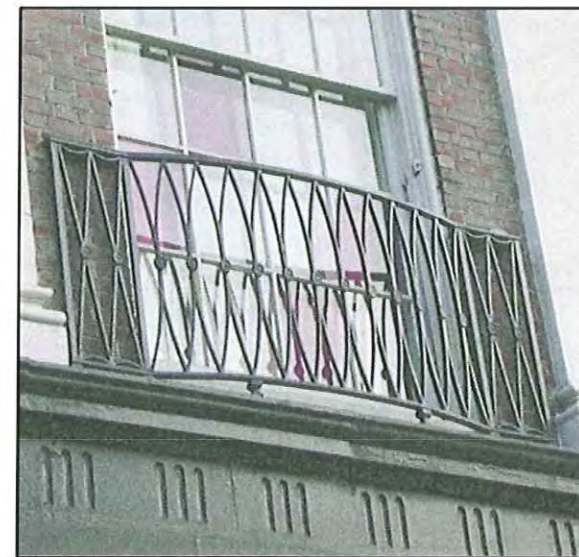
Painted Metal Railing
