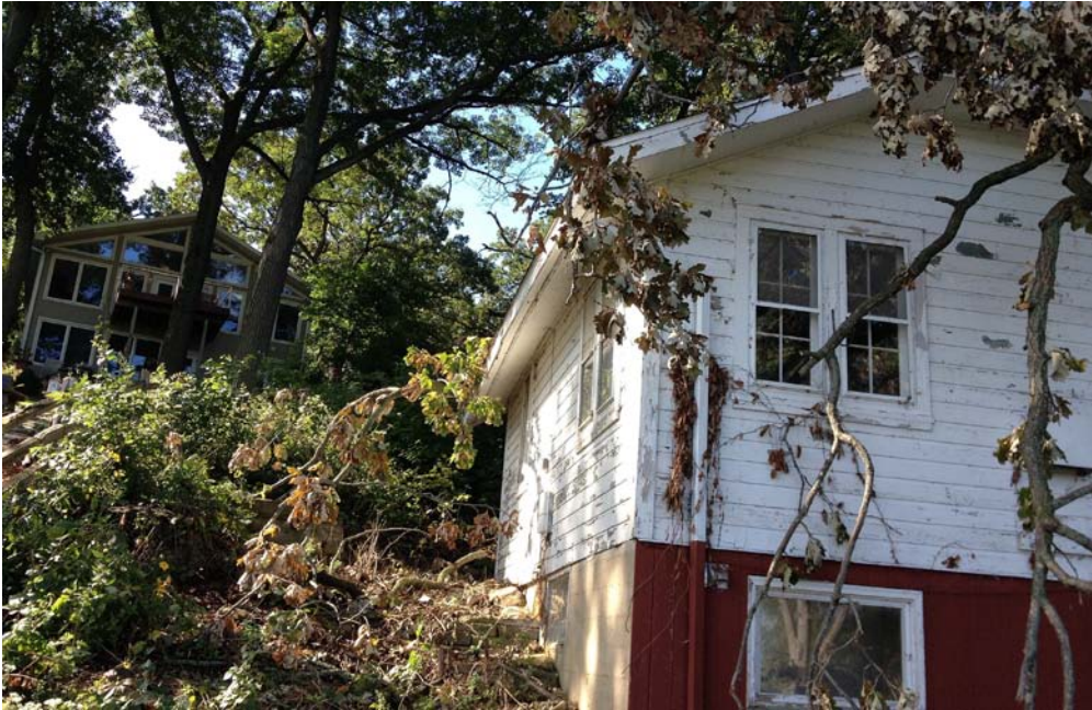
City of Madison photo of storm damage
