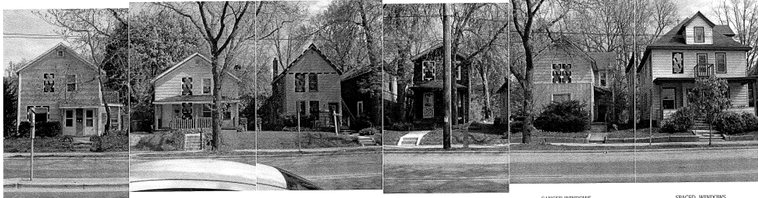
SPACED WINDOWS NARROW HORIZONTAL SIDING
