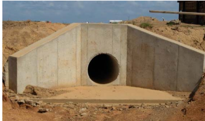
TYPICAL PIPE WITH NO SURFACE TREATMENTS
