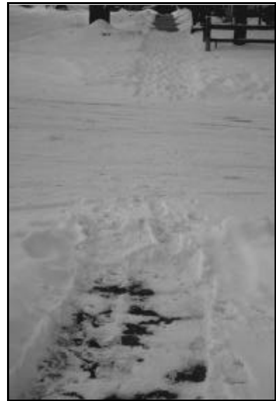
When snow has not been removed from sidewalks, pedestrian connectors, curb cuts, bus pads and medians, pedestrian travel is significantly impacted.
