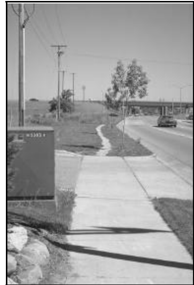
Worn ruts often develop adjacent to the roadway where sidewalks are not provided, indicating a demonstrated need.
