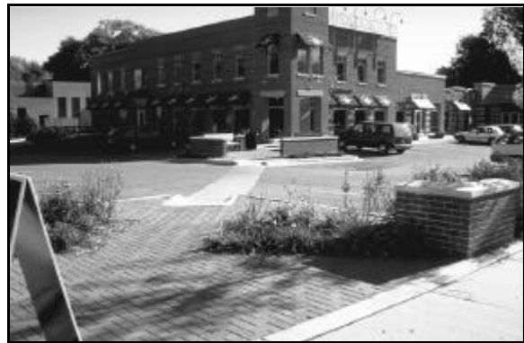
This short pedestrian connector across this parking lot enhances pedestrian access from the sidewalk network to Knickerbocker Place on Monroe Street.
