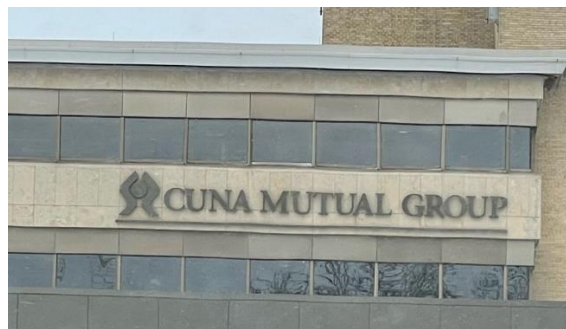
5810 Mineral Point Road – Approximately 90 sf2 THESE LETTERS HAVE BEEN REMOVED
