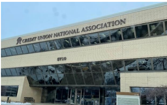
5710 Mineral Point Road – Approximately 134 sf2 THESE LETTERS ARE BEING REMOVED
