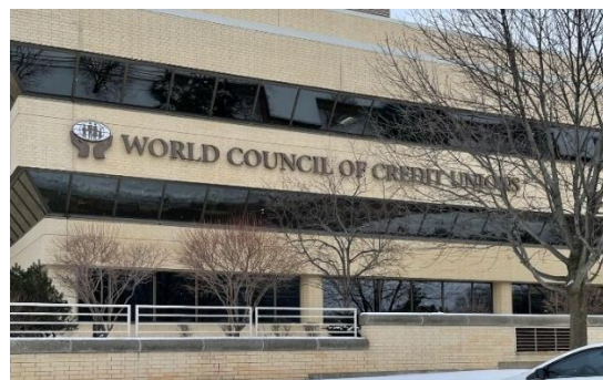
5710 Mineral Point Road – Approximately 139 sf2 THESE LETTERS ARE BEING REMOVED
