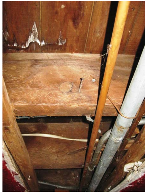
Photo 6 – 1 st floor joist framing
