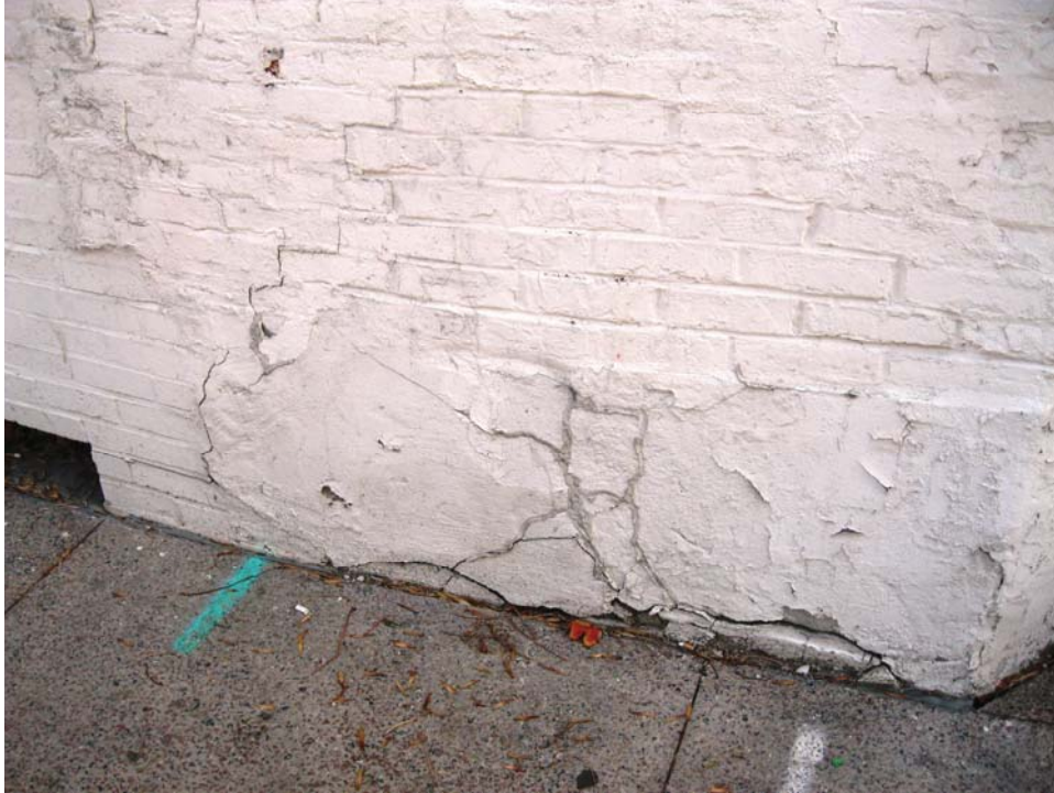
Photo 11 – Exterior wall base at Fairchild Street sidewalk
