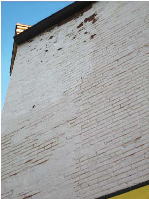
Photo 3 – Fairchild Street elevation at corner
