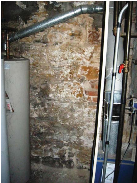
Photo 9 – Basement wall along Fairchild Street
