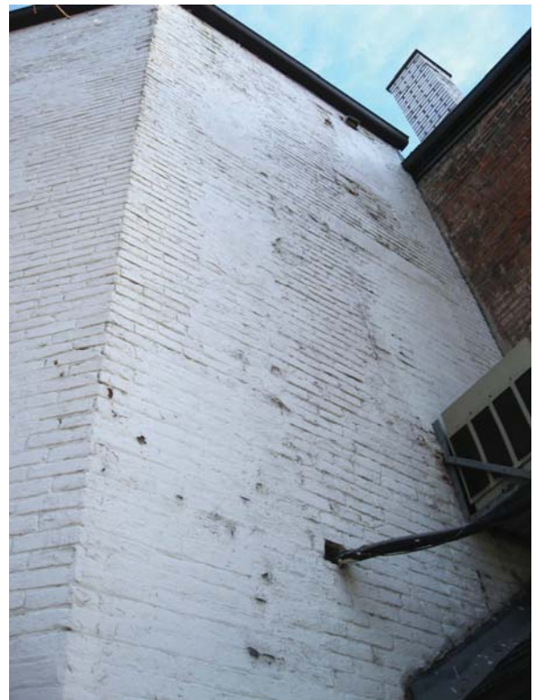
Photo 4 – Fairchild Street elevation at building rear
