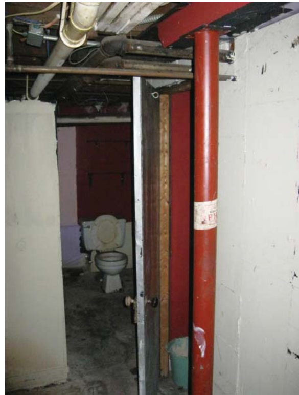
Photo 10 – 1 st floor shoring beam and post
