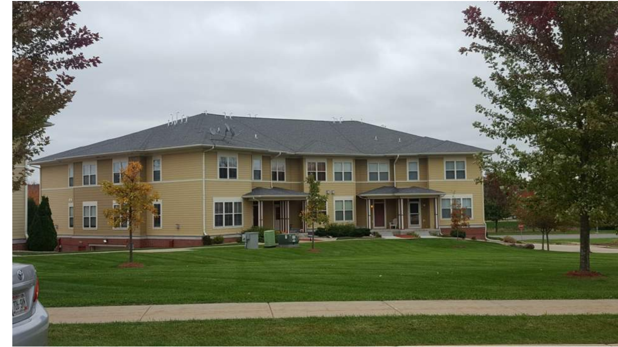
Rear of 9 Unit Building
