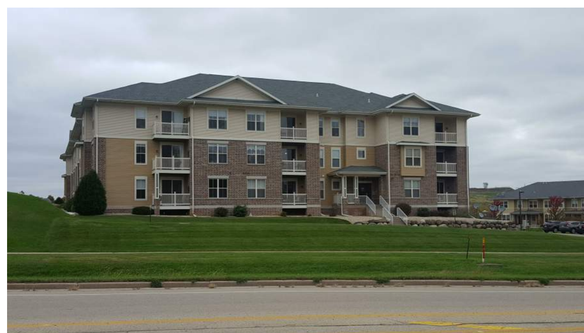
48 Unit Bldg from Nelson Rd. to N.
