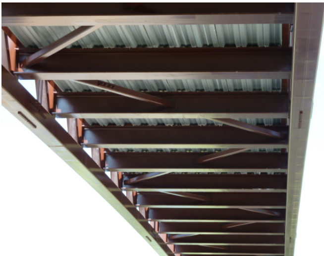
Under deck framing Bowstring truss
