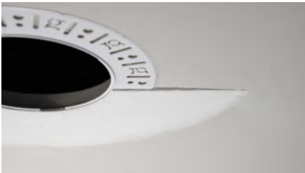
Partially finished mud ring, showing cross-section detail.
