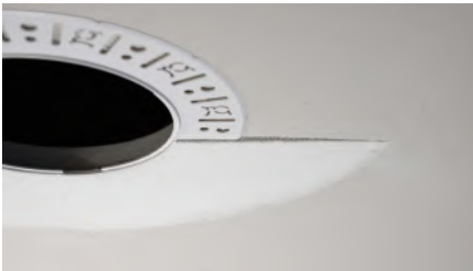
Partially finished mud ring, showing cross-section detail.
