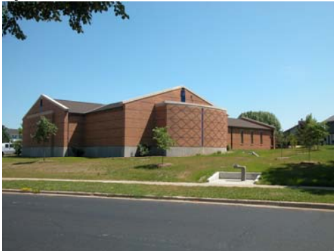
Outside View of Iron and Manganese Treatment System at Well 29
