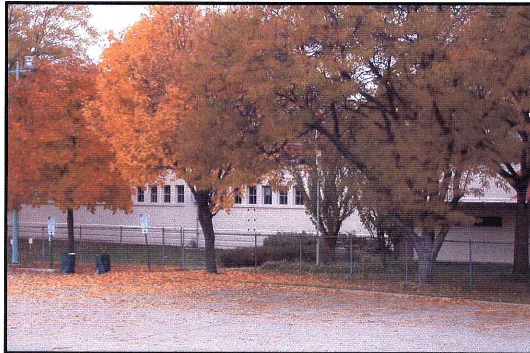
VIEW OF EXISTING MAINTENANCE FACILITY
