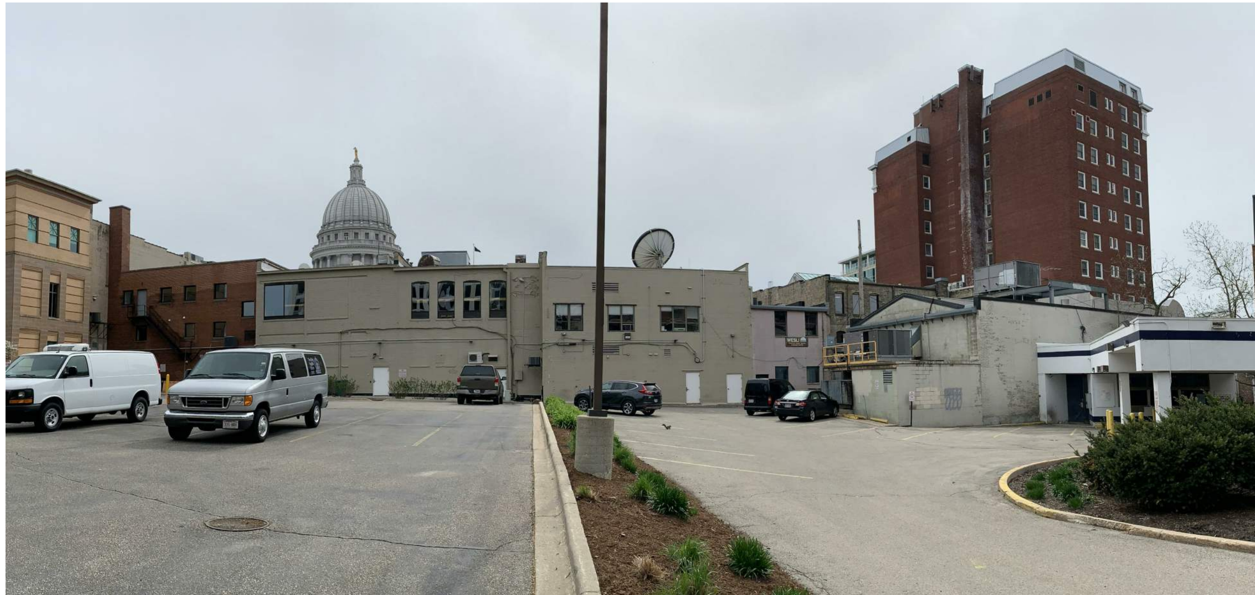
EXISTING CONDITIONS - OUTER LOOP
