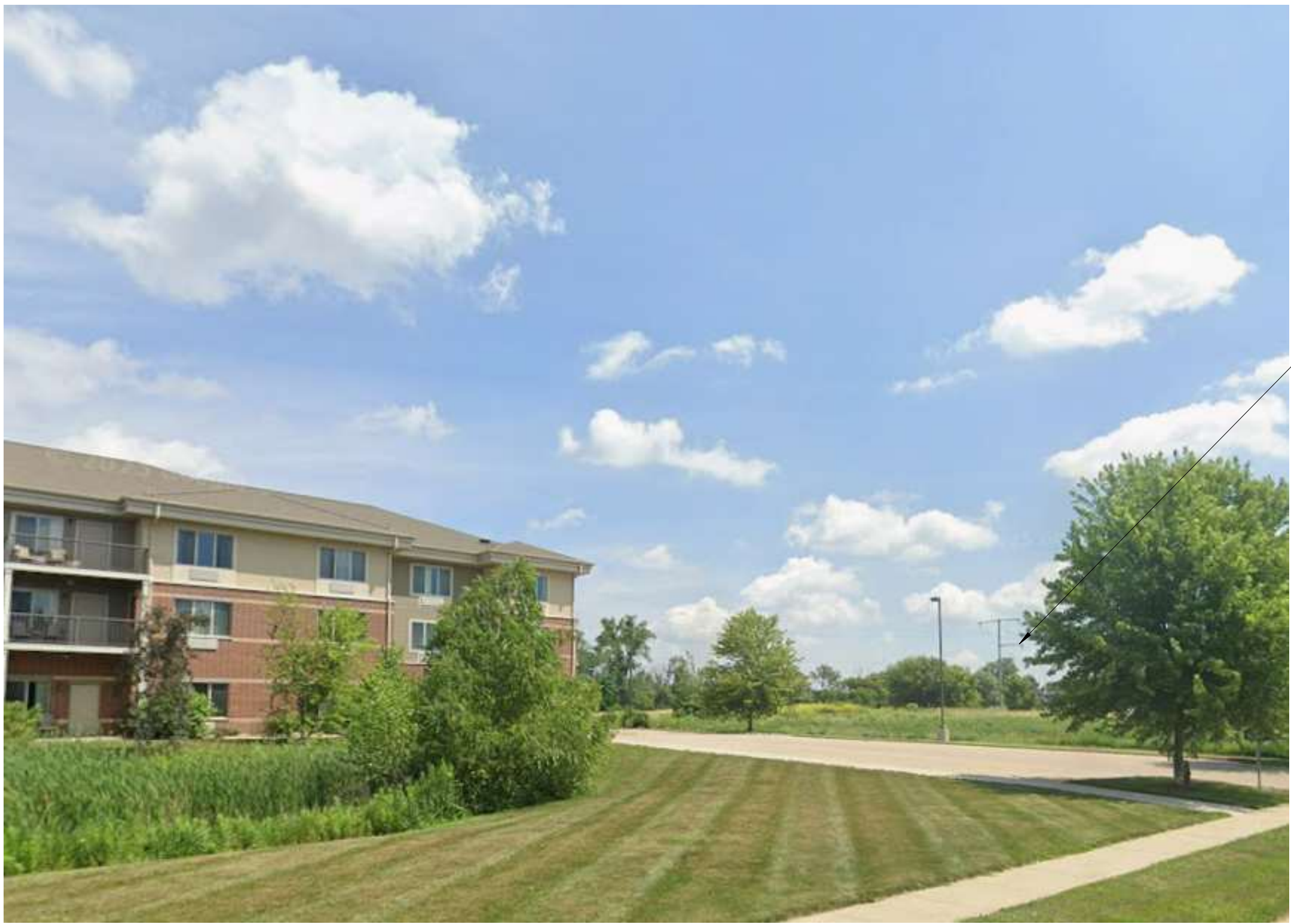
BUILDING ADJACENT TO PROPOSED BUILDING - WEST SIDE
