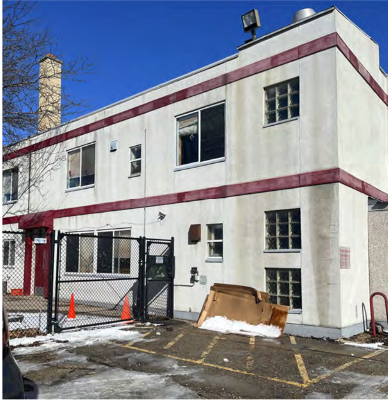
Photos of existing building to be removed – 654 Williamson
