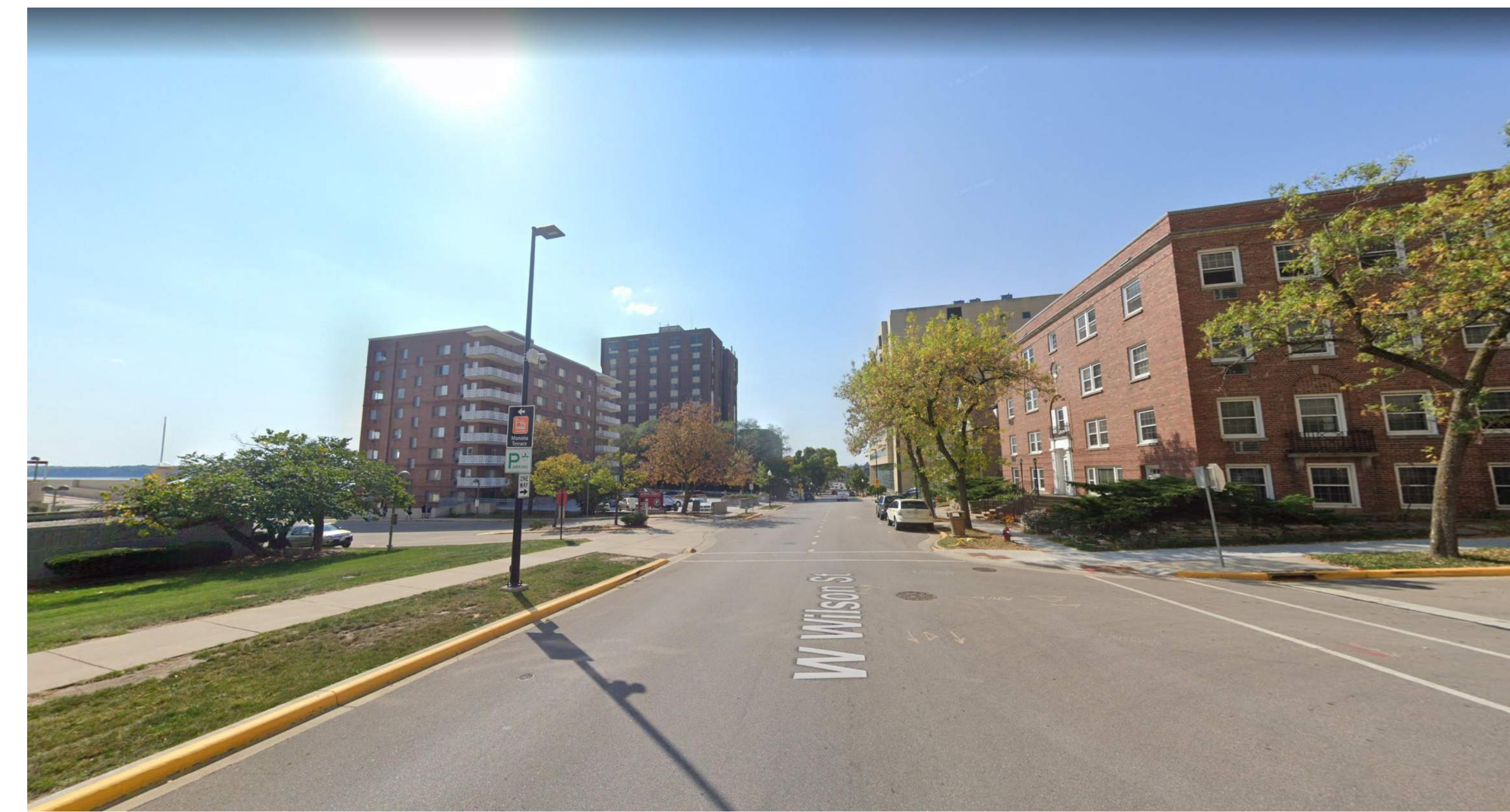
VIEW LOOKING SW ALONG WILSON STREET
