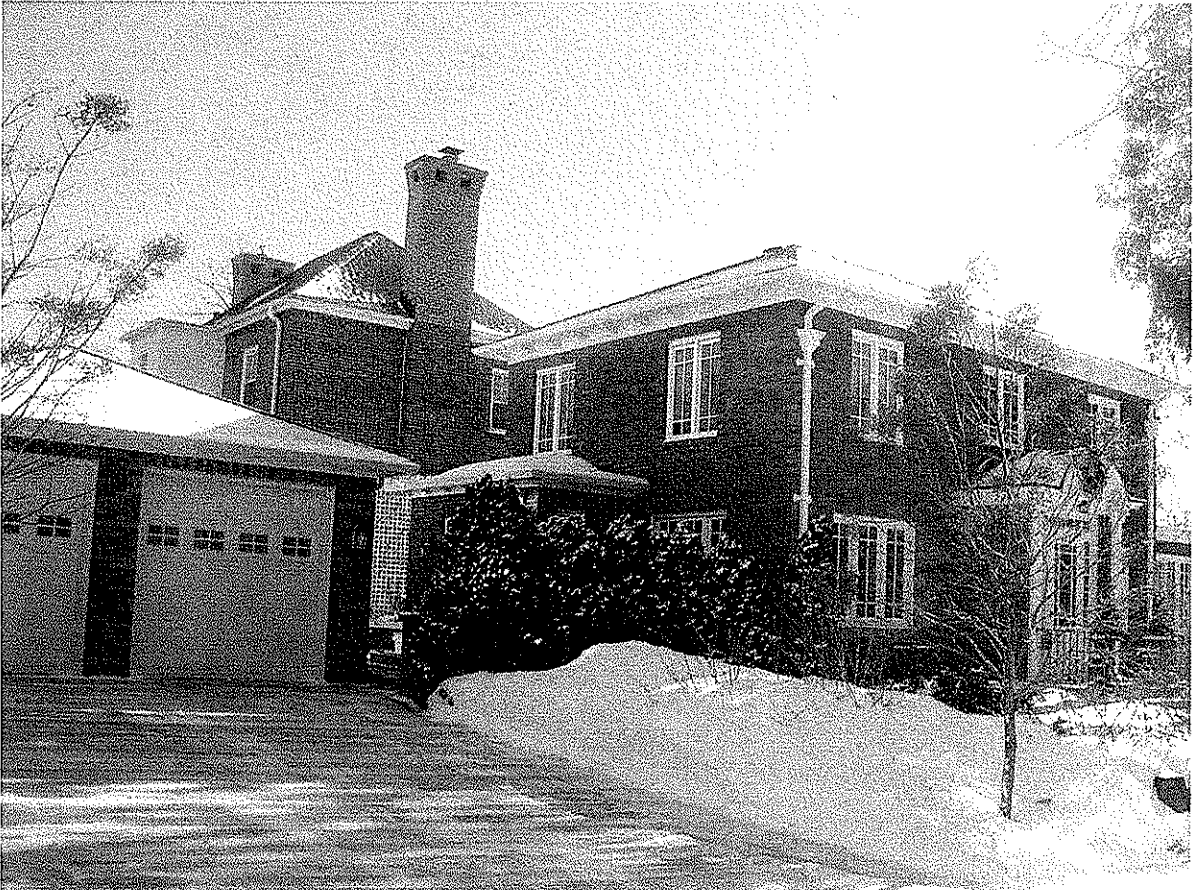
North west view of 207 North Spooner Street as viewed from driveway.
