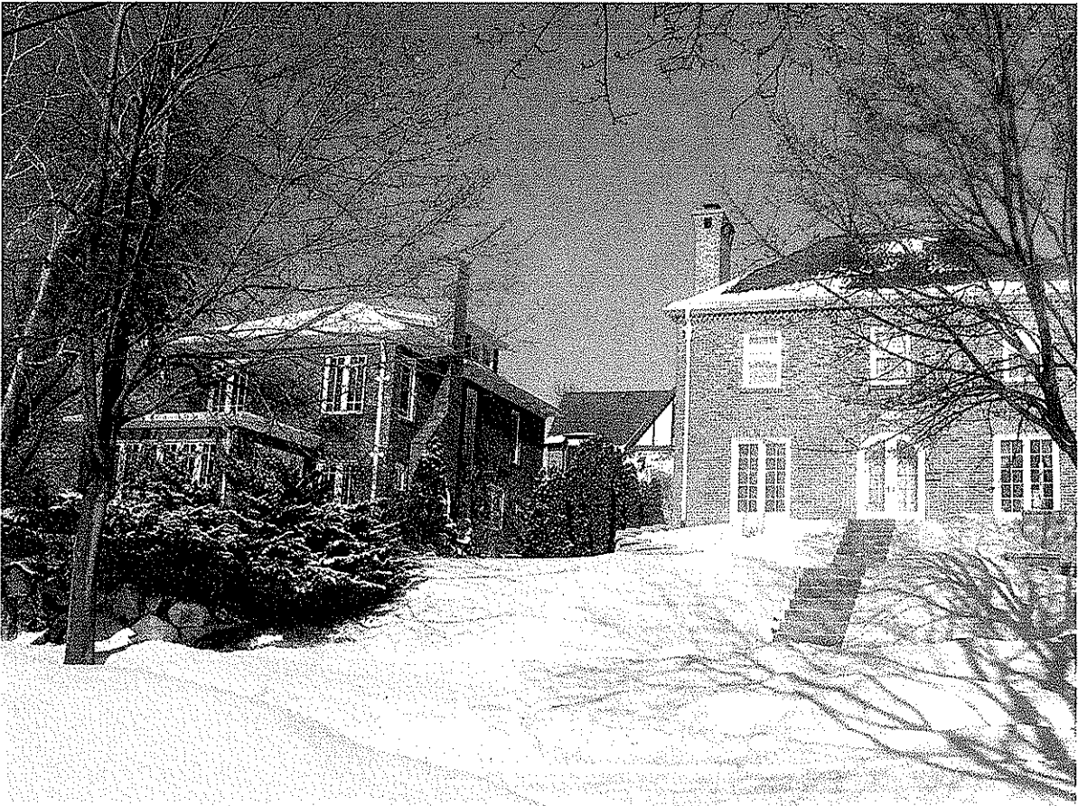
South elevation of 207 North Spooner Street & 1722 Summit Avenue.
