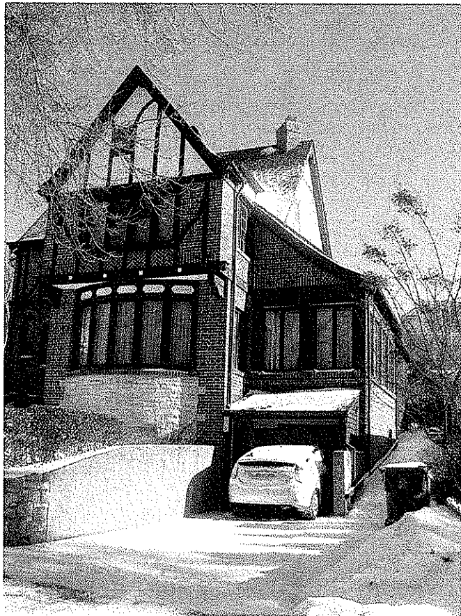
209 North Spooner Street. Immediately adjacent north neighbor.
