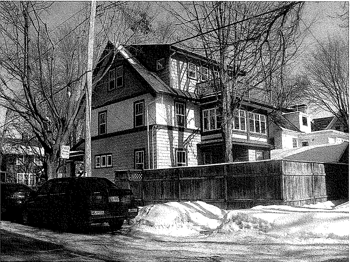
Rear of 1725 Chadbourne Avenue. Previously approved by Landmarks Commission.
