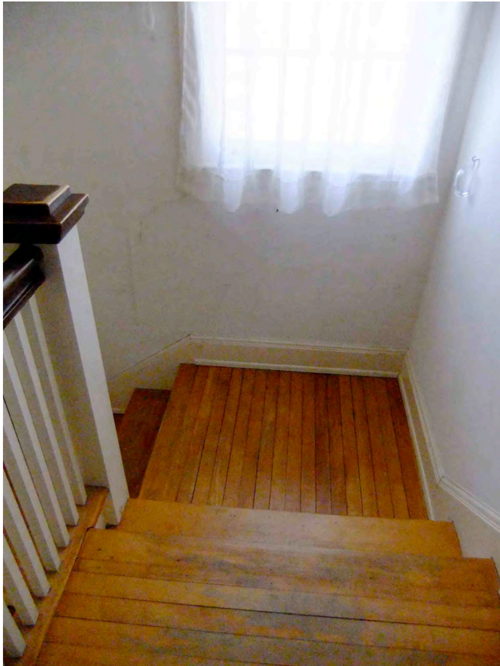
Stairwell (faces North)
