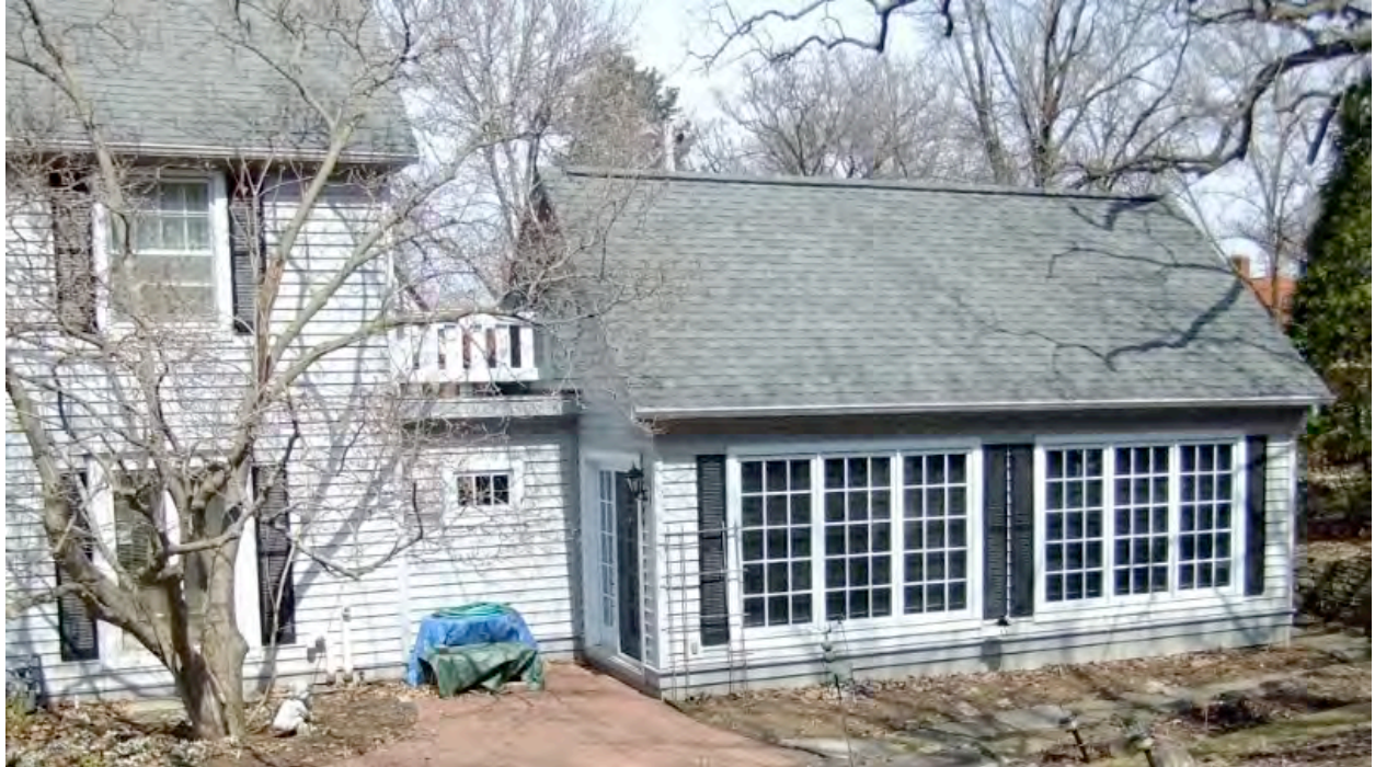
South Elevation – Garden Room (does not face a street)
